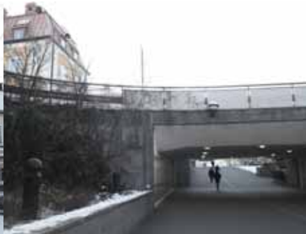
Walking tunnel to railway station.
