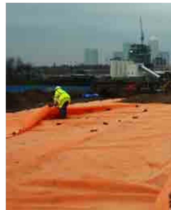
Orange geotextile was used in London when building for the Olympic Games in 2012. The soil underneath is heavily contaminated and radioactive (Photo: Games Monitor).
