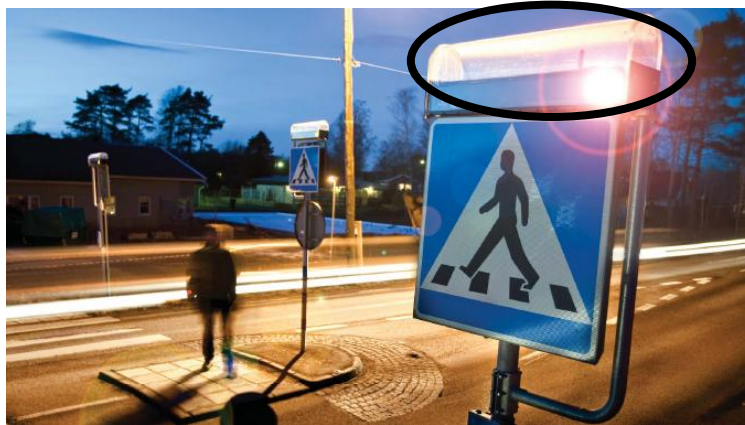
Figure 4. An example of an infrastructure-based active safety system. A road sign is equipped with a light-emitting device that is activated when pedestrians are in the vicinity of the zebra crossing. Courtesy of Amparo Solutions AB.
