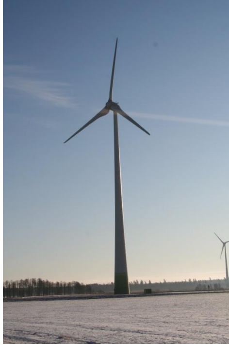
Figure 29: Enercon E-53 wind turbine
