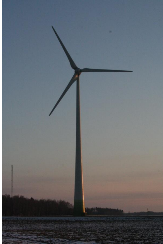
Figure 11: Enercon E-82 wind turbine
