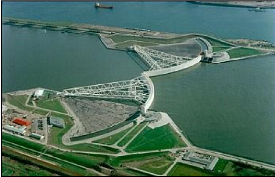
Figure 13: The Maeslant barrier in Rotterdam, Netherlands 9
