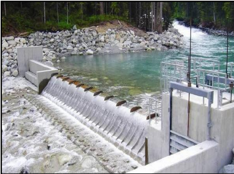
Figure 11: The Coanda diversion structure 6
