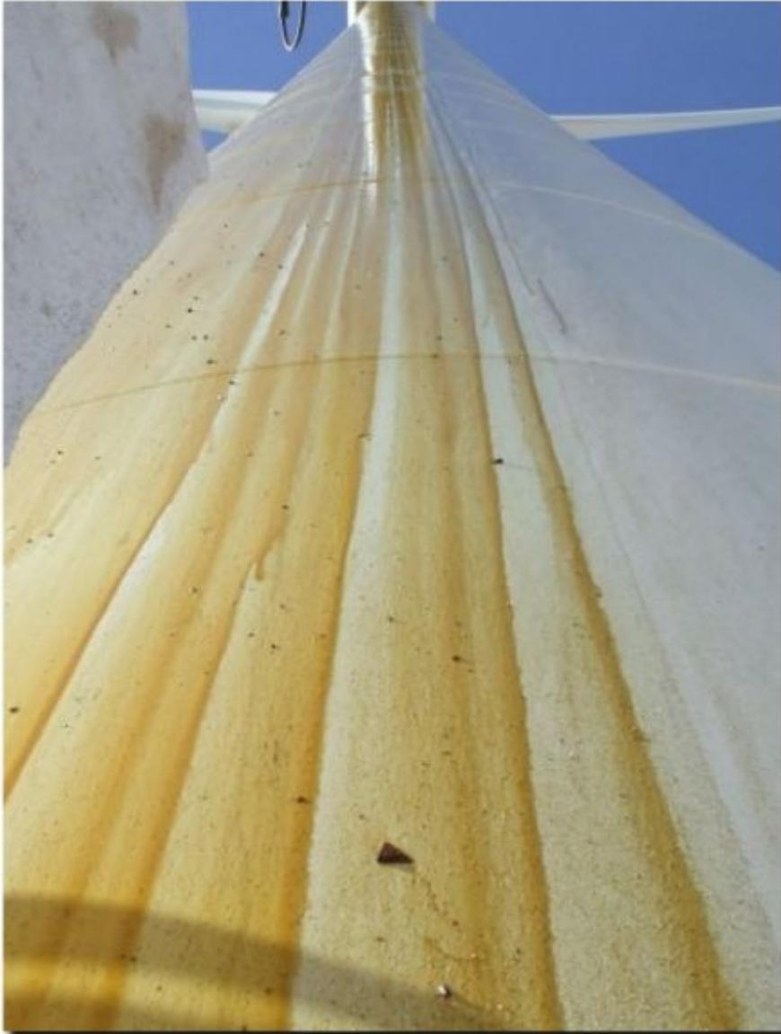
Photo of oil leakage from wind power plant. Source:
