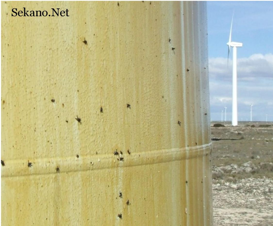
Photo of oil leakage from wind power plant. Source:
