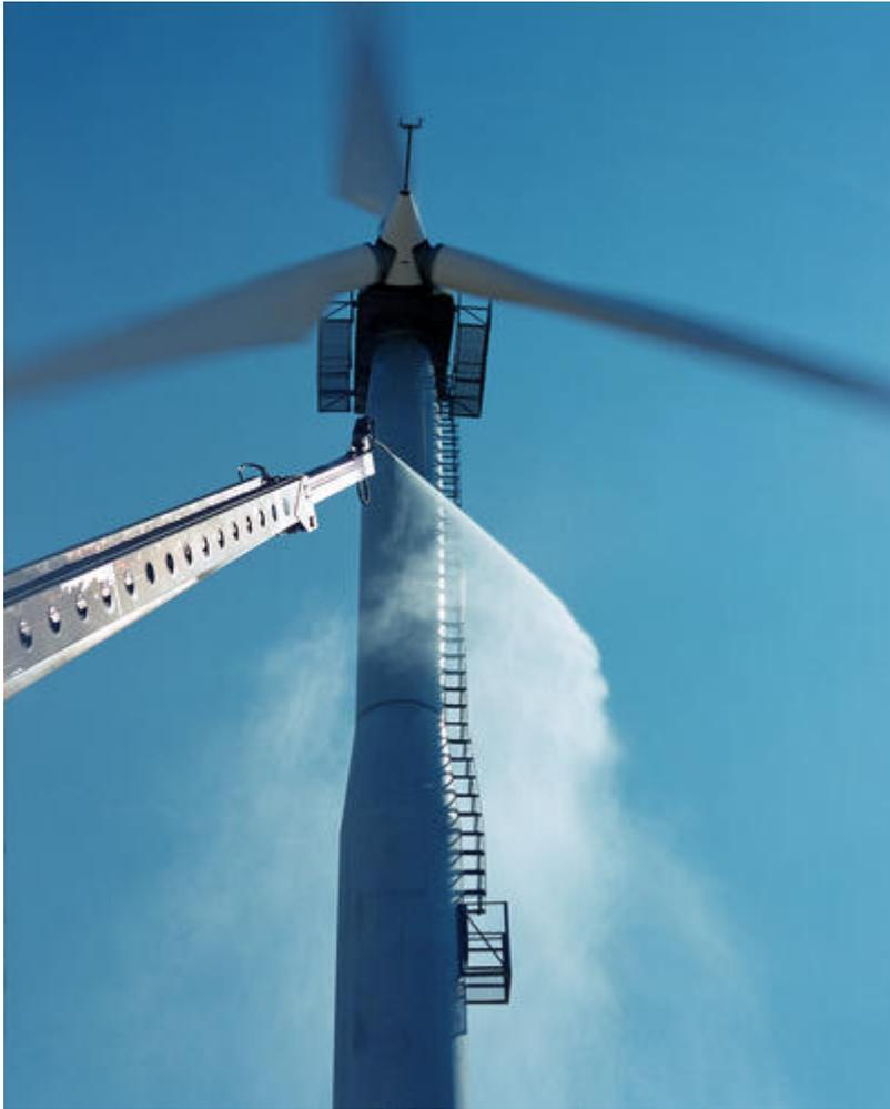
Photo of washing of a wind power plant. Source:
