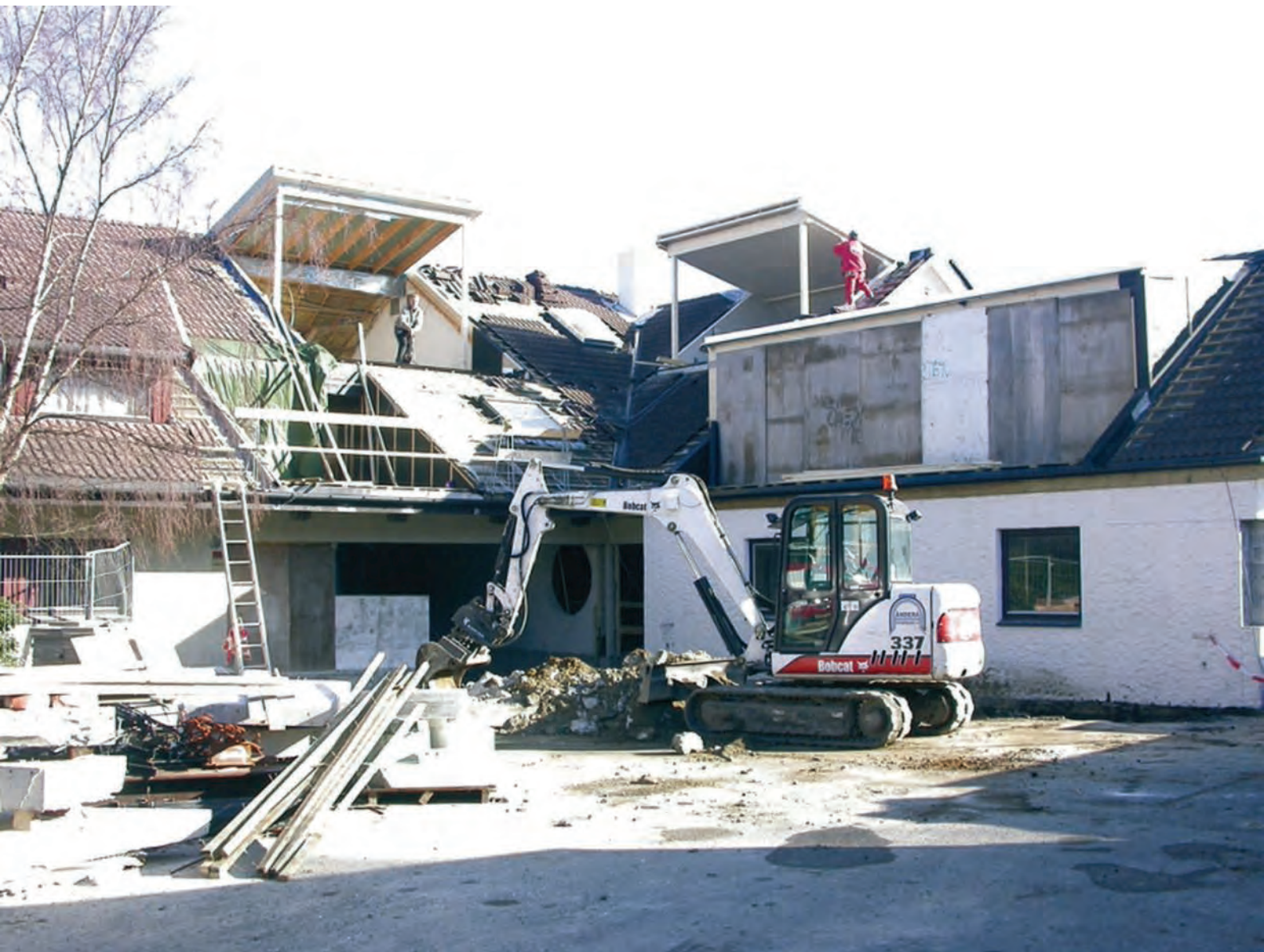
Pic 5: Construction photo. The roof was lifted and opened for terraces. © H&H
