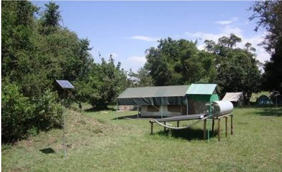
Figure 8 Solar panel and solar collector is used to support a small camp in rural Kenya with power and hot water.
