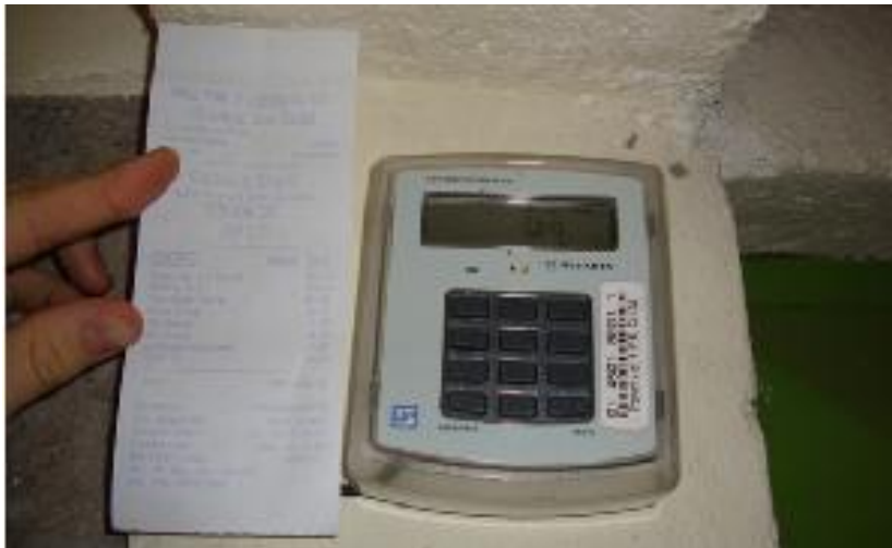
Figure 6 Electricity meter for pre-paid electricity bill.
