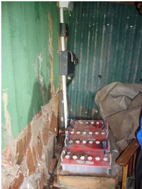
Figure 14 Lead-Acid batteries and a charge regulator used for a small solar power system.
