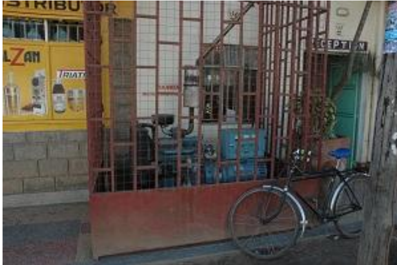
Figure 7 Diesel generator at a hotel used to prevent power blackouts from the electricity grid.
