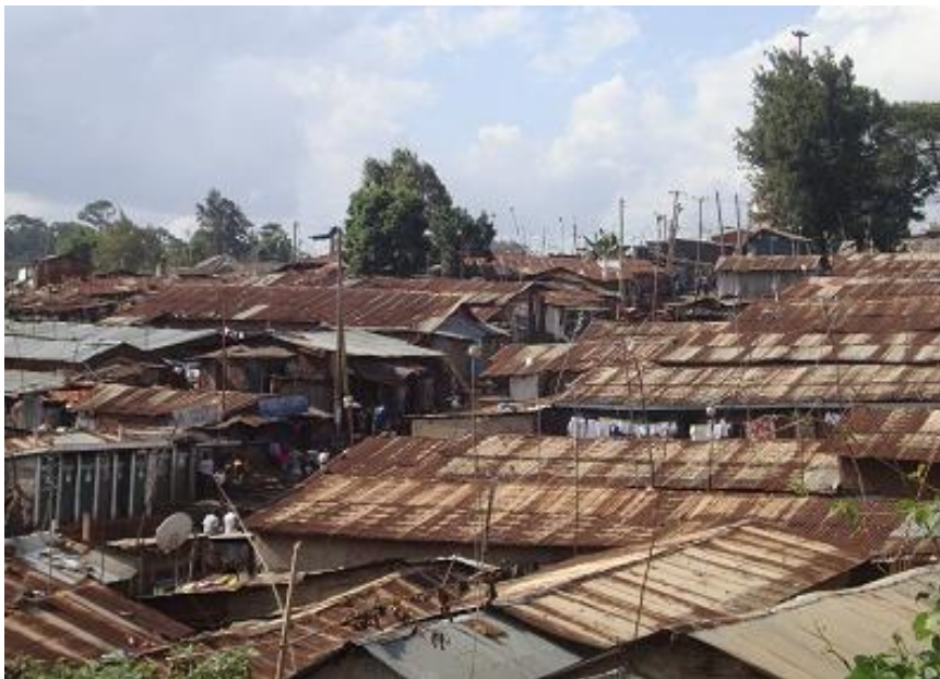
Figure 2 Most dwellings in Nairobi are connected to the electricity grid.
