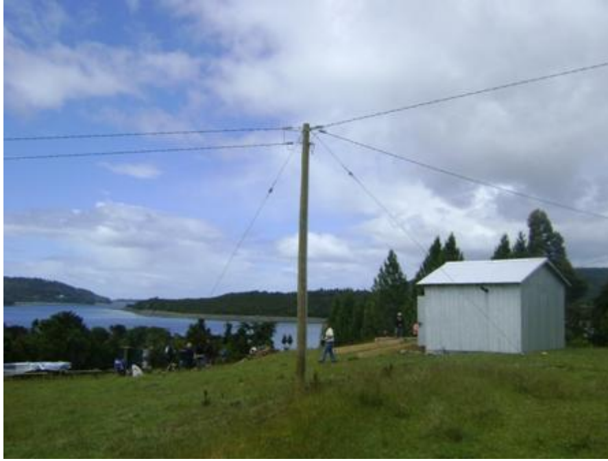
Figure 4: Newly installed electricity grid on the island of Cheniao, Municipality of Quemchi. The system was inaugurated the 7 th of December of 2010.
