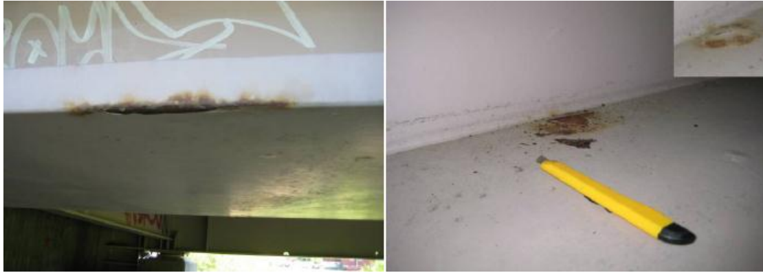
Figure 7.47 On the left side rust damage occurred and on the right side rust blisters occurred [19].
