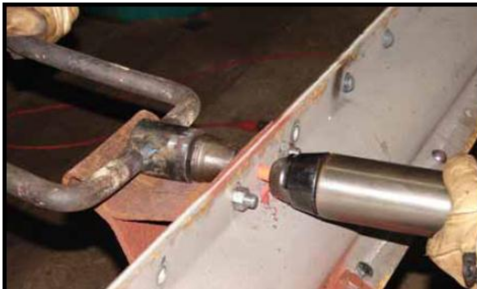
Figure 6.6 The second rivet heat is shaped [15].
