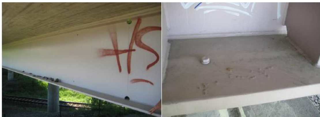
Figure 7.46 On the left side graffiti and stones can be seen and on the right side rust blisters can be seen [19].
