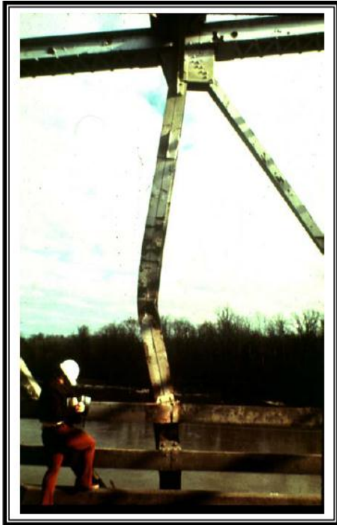
(a) Category W damage on a built-up double channel truss member. The damage was caused by a log falling from a truck on a bridge in North Louisiana.
