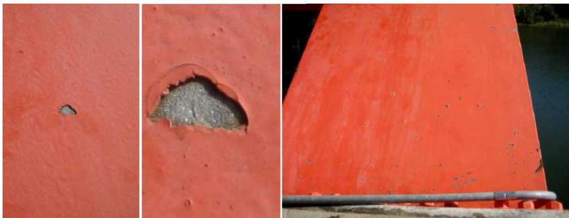
Figure 7.51 Dirty components causing corrosion [19].
