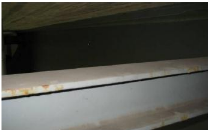
Figure 7.41 Rust created on cross-beam [19].
