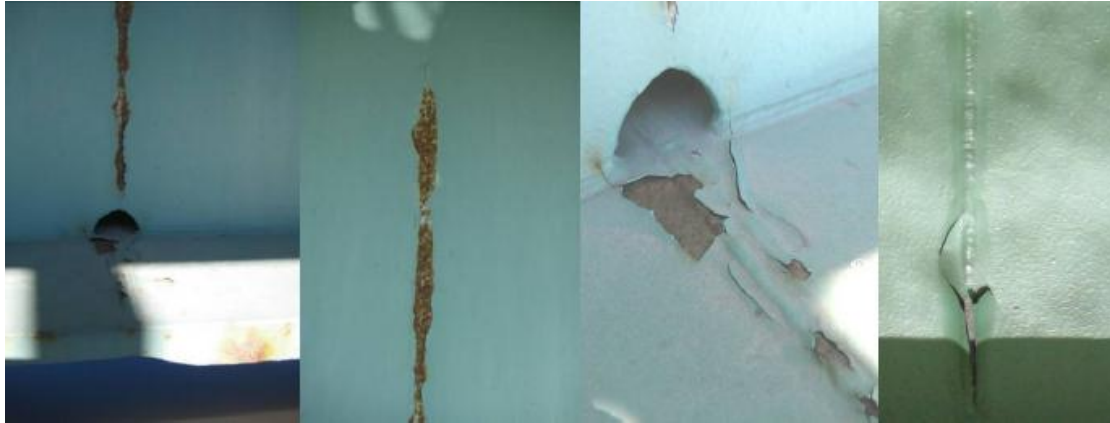
Figure 7.44 Paint flaking and rust created on main welds [19].
