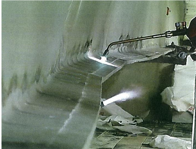
Figure 7.24 Straightening work of damaged beam [3].
