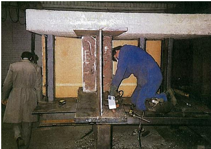
Figure 7.1 A mock-up was built before the operation [3].
