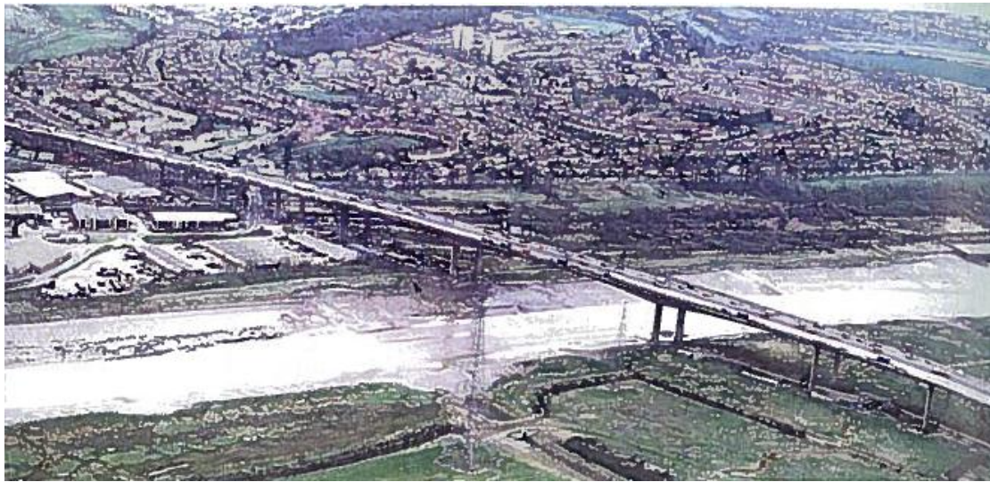
Figure 7.19 A view of Avonmouth Bridge [3].
