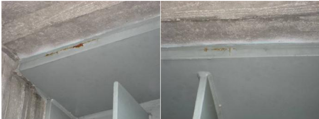
Figure 7.40 Rust created between the top flange and concrete [19].
