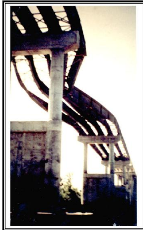
(b) Category W damage to main girders during construction of a Louisiana bridge.
