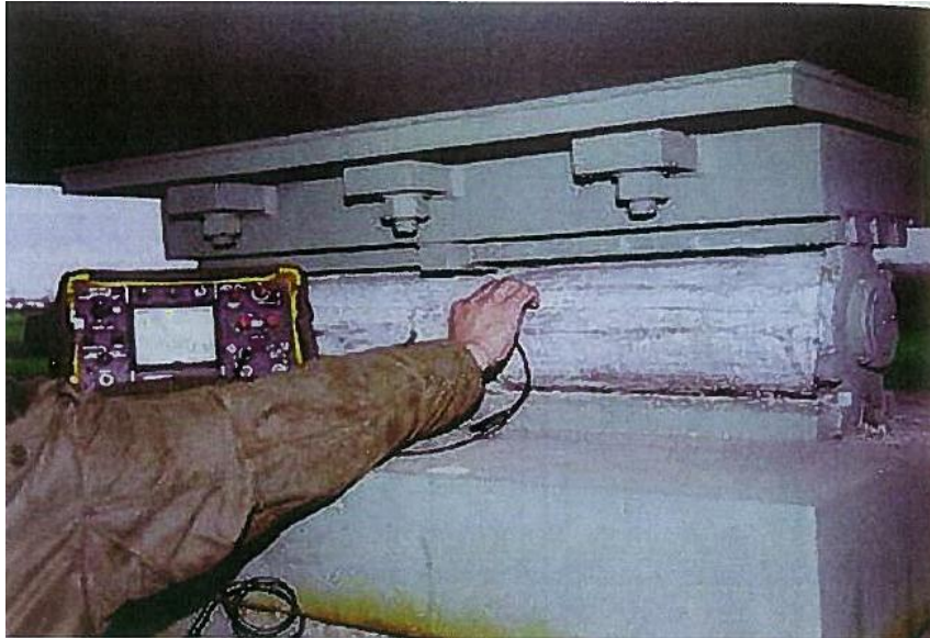
Figure 7.5 The damaged rolling bearing [3].
