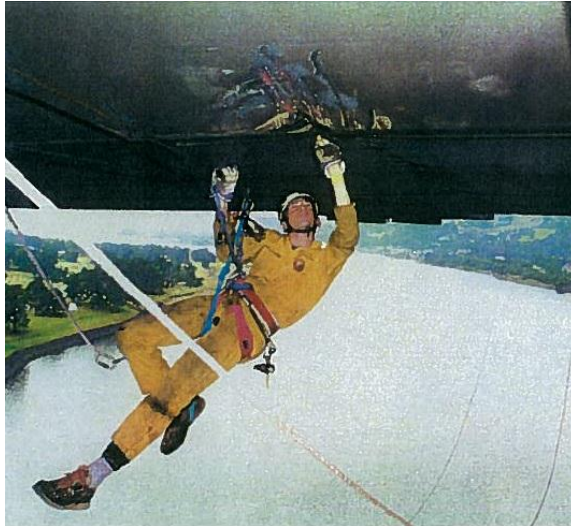
Figure 7.26 Damage caused by a collision [3].
