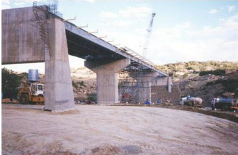
Figure 4.3 Erection of continuous steel beam bridge (place and name of the bridge are unknown) [18].
