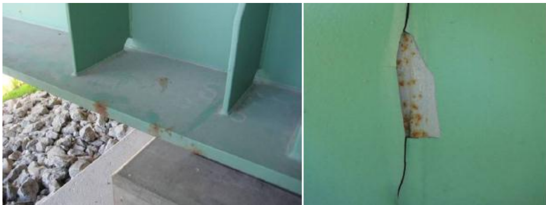
Figure 7.42 On the left side rust created on bottom flange and on the right side cracked paint, paint flaking and rust in main beam can be seen [19].
