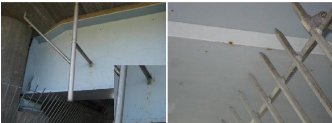
Figure 7.33 Damage from stone throw and rust on bottom flange, East abutment [19].
