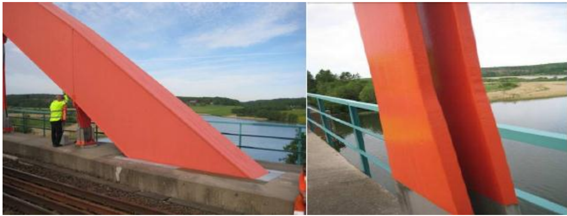
Figure 7.49 Bottom part of the arch was re-constructed and stainless steel used [19].
