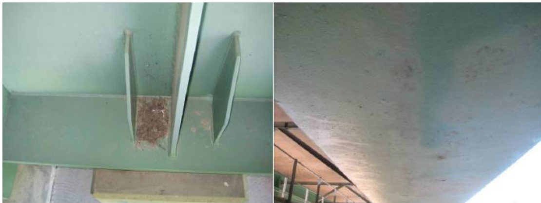
Figure 7.43 A roost and rust in bottom flanges [19].
