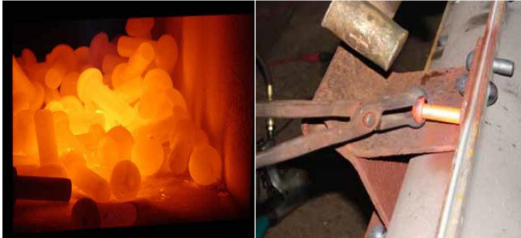
Figure 6.5 Heating of the rivets and introducing the holes [15].
