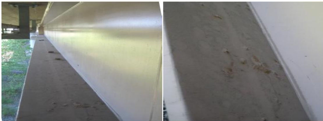
Figure 7.48 Rust damages on bottom flange [19].
