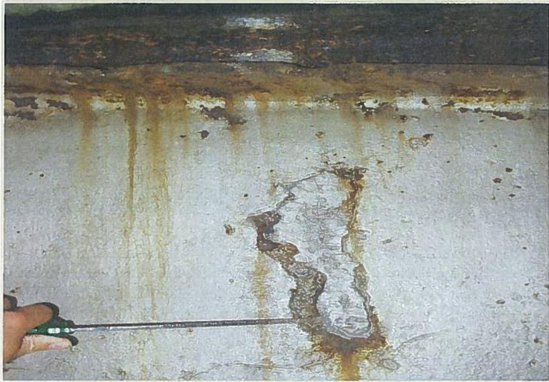
Note the corrosion staining to the ironwork
