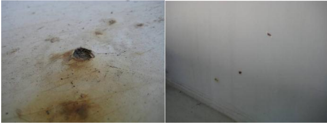
Figure 7.55 On the left side deep-seated rust can be seen and on the right side stone throw damages can be seen [19].
