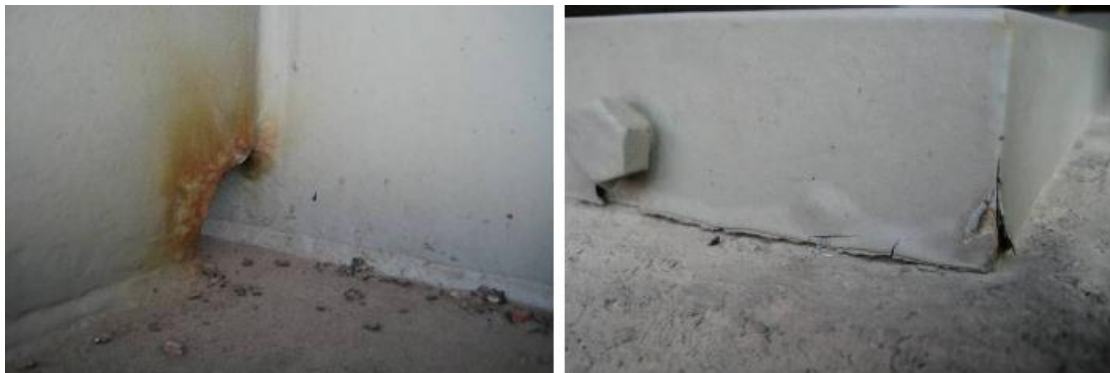
Figure 7.37 On the left side rust created on a notch and on the right side paint of the bearing loosened (in N abutment) [19].
