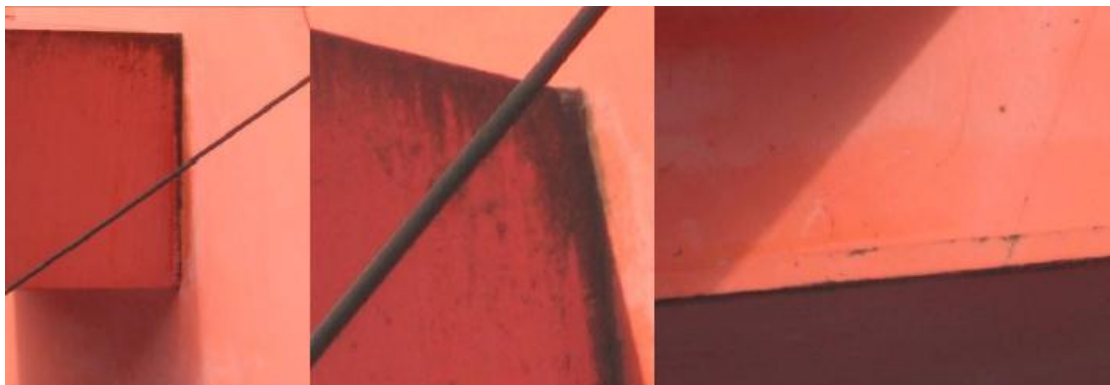
Figure 7.51 Dirty components causing corrosion [19].
