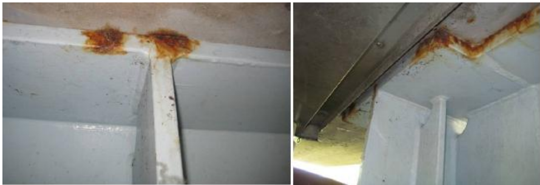
Figure 7.35 On the left side rust detected on top flange against concrete and on the right side rust occurred on splice [19].
