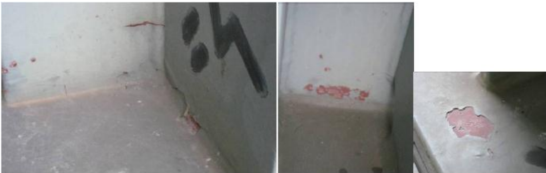
Figure 7.29 Flaking of painting, S abutment [19].
