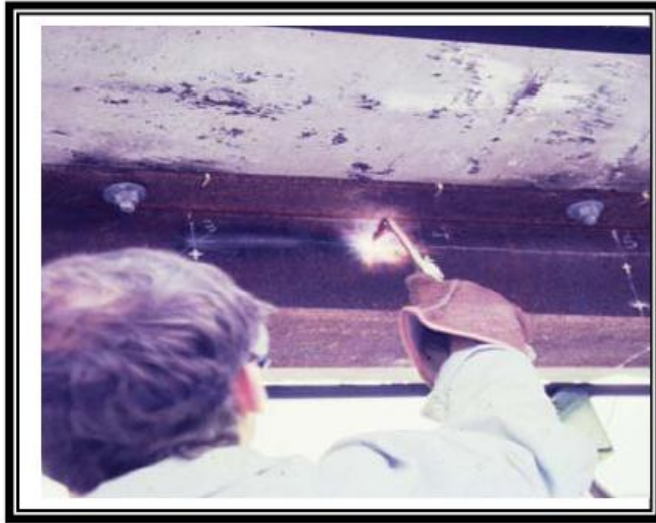
Figure 6.18 Line heating in the web [11].
