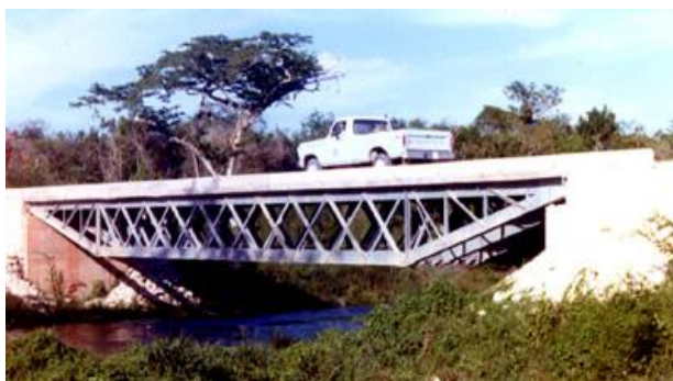
Figure 4.5 Steel over truss bridge in Belize (name of the bridge is unknown) [18].
