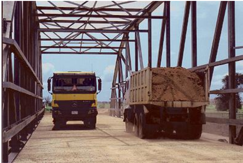
Figure 4.10 Trough truss bridge (name and place of the bridge are unknown) [18].
