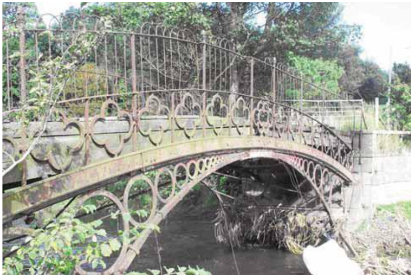
Figure 2.3 Cast iron after 50 years without maintenance, corrosion is evident [1].
