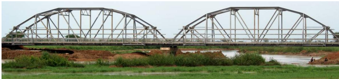
Figure 4.16 Steel bowstring girder bridge in Sudan [18].
