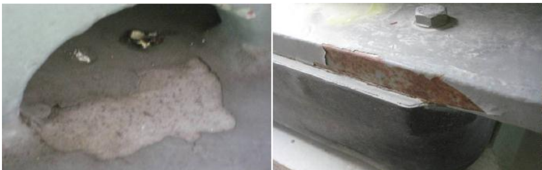
Figure 7.31 On the left side flaking of painting next to a notch in S abutment and on the right side flaking of bearing painting in N abutment [19].
