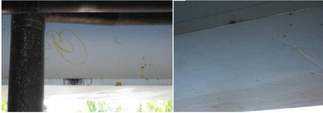
Figure 7.34 Rust on the main beam [19].
