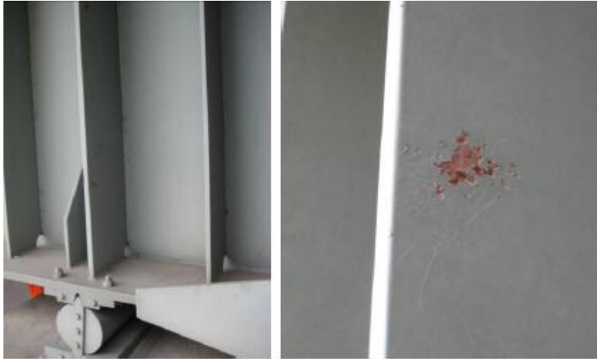
Figure 7.39 Detected damage on stiffener [19].
