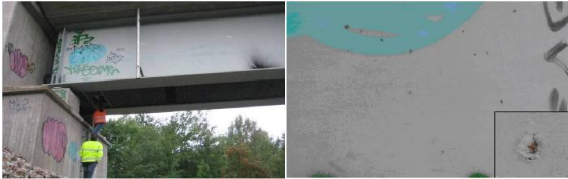
Figure 7.28 S and N abutments, on the right side graffiti can be seen and on the left side damage from stone can be seen [19].
