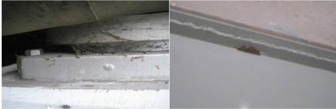
Figure 7.32 On the left side a blowhole without rust in S and N abutment and on the right side a rust under painting [19].
