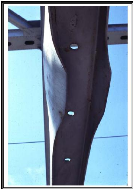
Category L damage showing flange buckles on wind bracing on Mississippi River Bridge in Greenville, MS.
