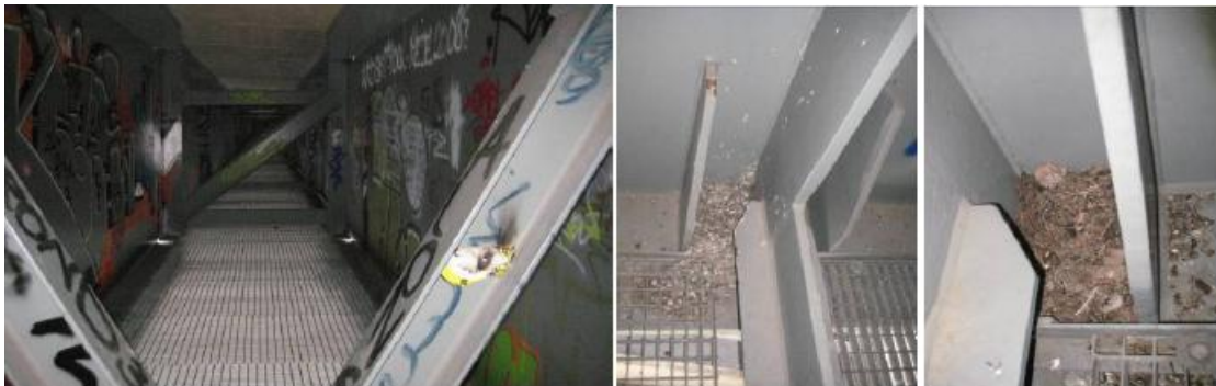
Figure 7.30 Graffiti and a roost inside of the bridge [19].
