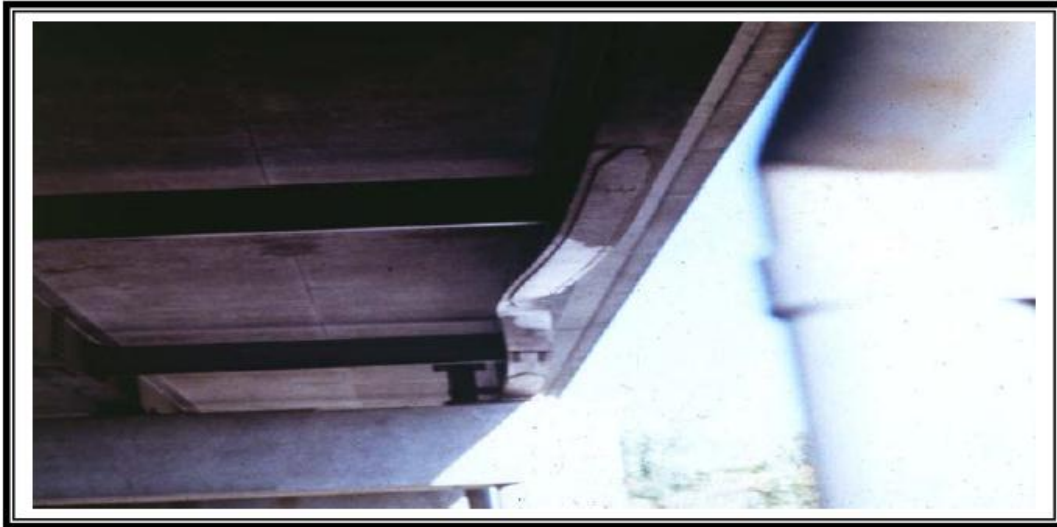
Category T damage on a composite bridge girder impacted by an over-height vehicle in Wisconsin.
