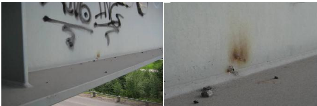
Figure 7.38 Graffiti, stone throw and rust [19].
