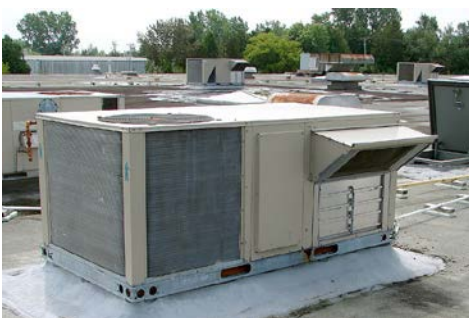
Figure 5: Package rooftop unit
