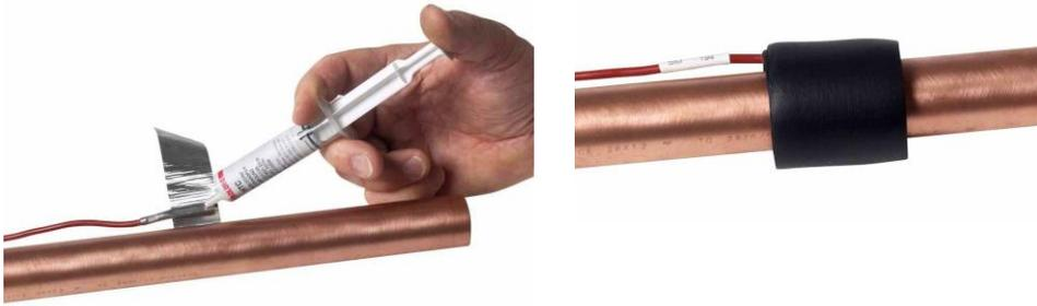
*Figure 3.9: Climacheck temperature sensor recommended set up*
