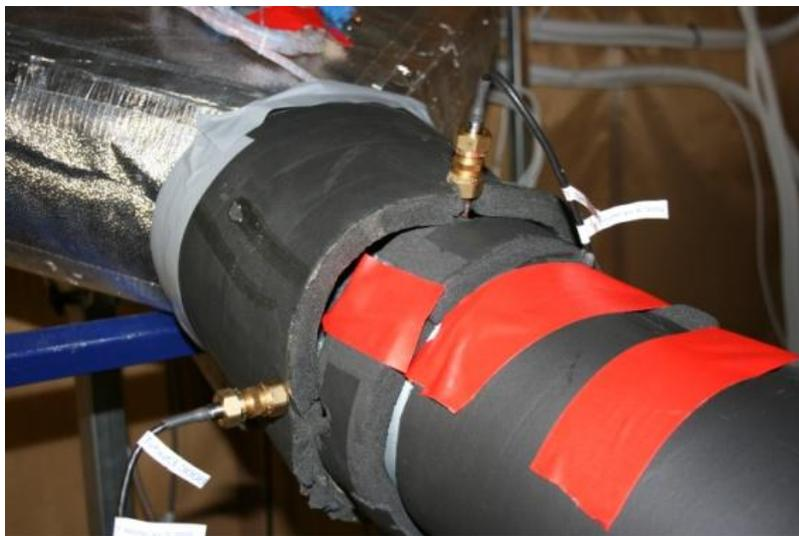
Figure 4.12: Temperatures sensors at the air outlet of the indoor unit (the SP Method)
