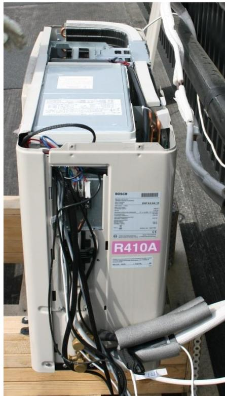
*Figure 4.16: On the bottom-left of the picture temperature sensors under the insulation (the Climacheck Method)*
