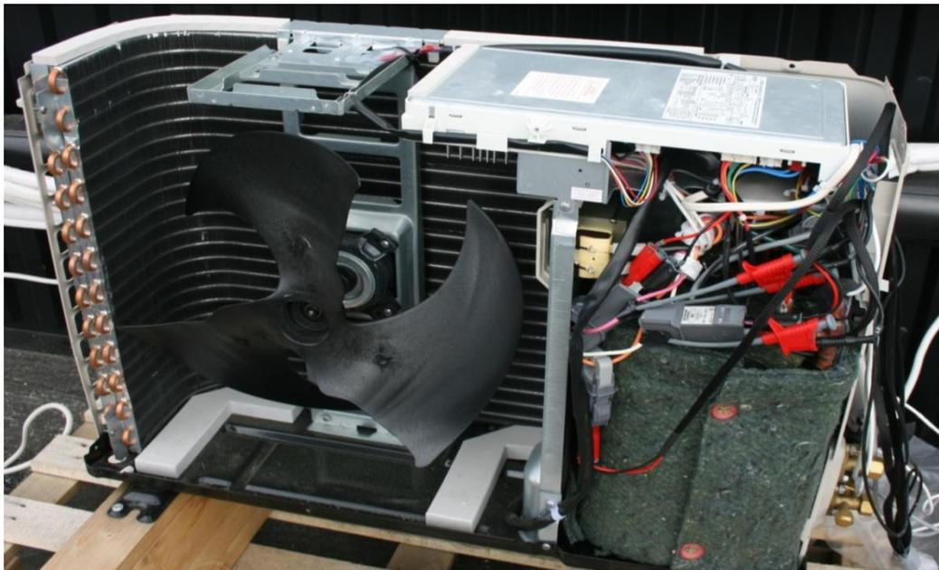
*Figure 7.1: Outlook of how Climacheck current clamps are installed*
