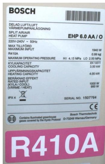
Figure 4.3: Heat pump properties as listed on the outdoor unit label
