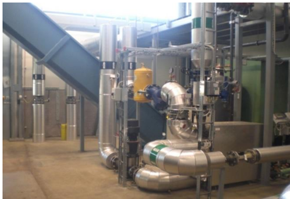
Figure 11 - Solar Hex and Solar loop forward/return pipes
