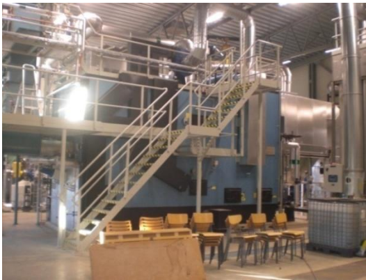
Figure 9 - Wood chip boiler
