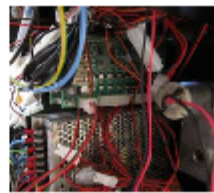
Figure 2. The observed circuitboards of the back.
