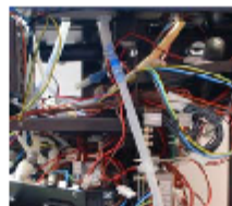
Figure 6. Cables spread all over the bottom of the machine. Less cables used and an easier removal of cables is preferred.
