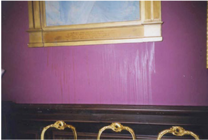
Figure 6.10 Condensed moisture running down the wall from behind one of several painting at the Renwick Gallery of the Smithsonian Institution in Washington, D.C. (Photograph courtesy of Ehrenkrantz, Eckstut & Kuhn, Architects)(Mecklenburg, 2007).
