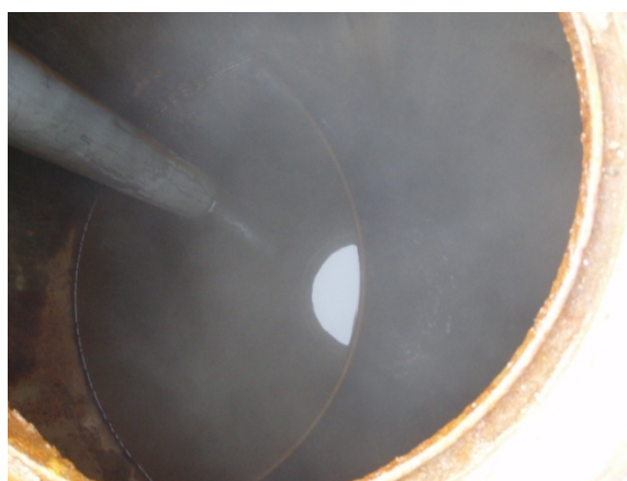
Figure 14 Reservoir of pit BZN-1 has higher water level, when reservoir has reached the maximum water level, it will flow over weir dam.
