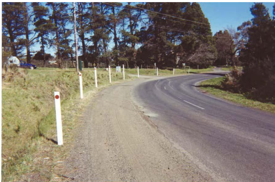
Figure 10 Curve countermeasure adding guide posts to reduce speed (Macaulay, et al., 2004)
