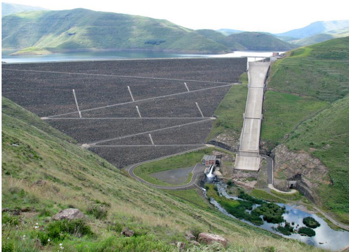
Figure 2.1 Downstream view of the Mohale dam in Lesotho
