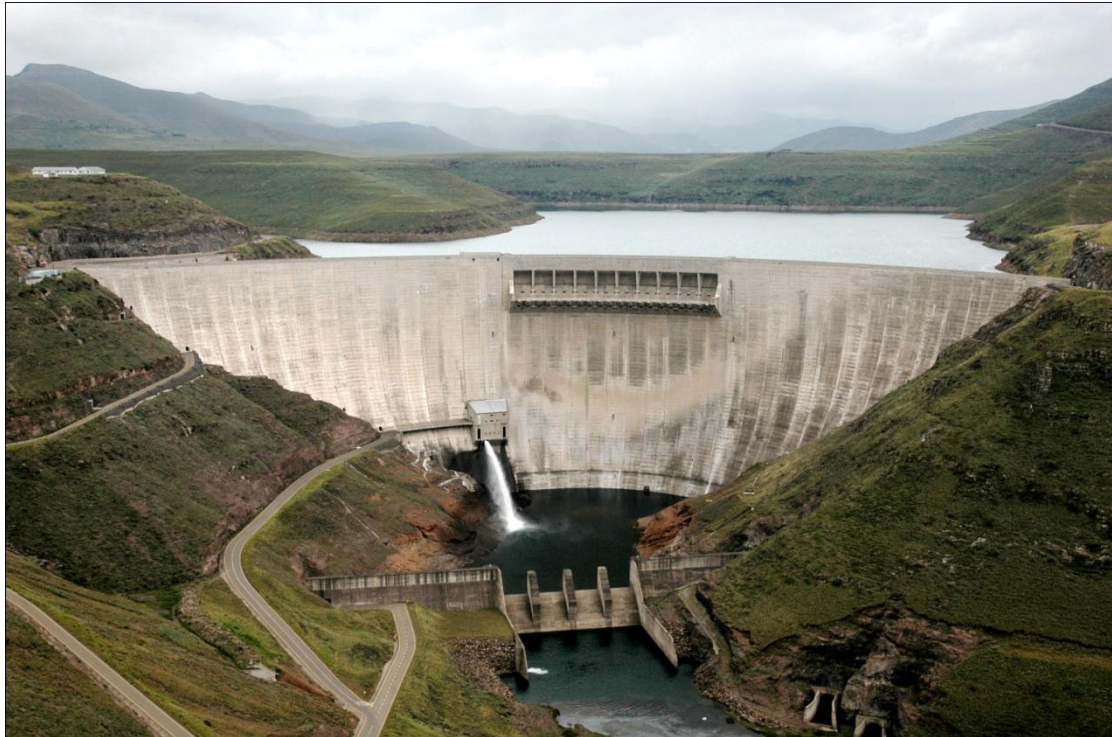
Figure 4.5 Recommended spillway design. Example of splitter spillway at Katse dam in Lesotho.
