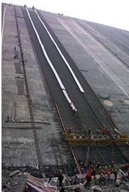
Figure 2.4 Placement of face concrete at Shuibuya dam in China.
