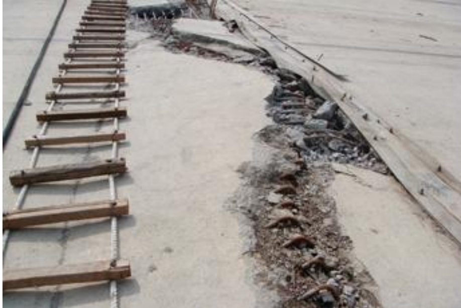
Figure 2.12 Damage along the vertical joints at Zipingpu dam in China due to earthquake.
