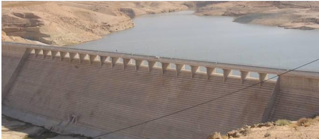
Figure 2.13 Downstream view of the Mujib dam in Jordan.
