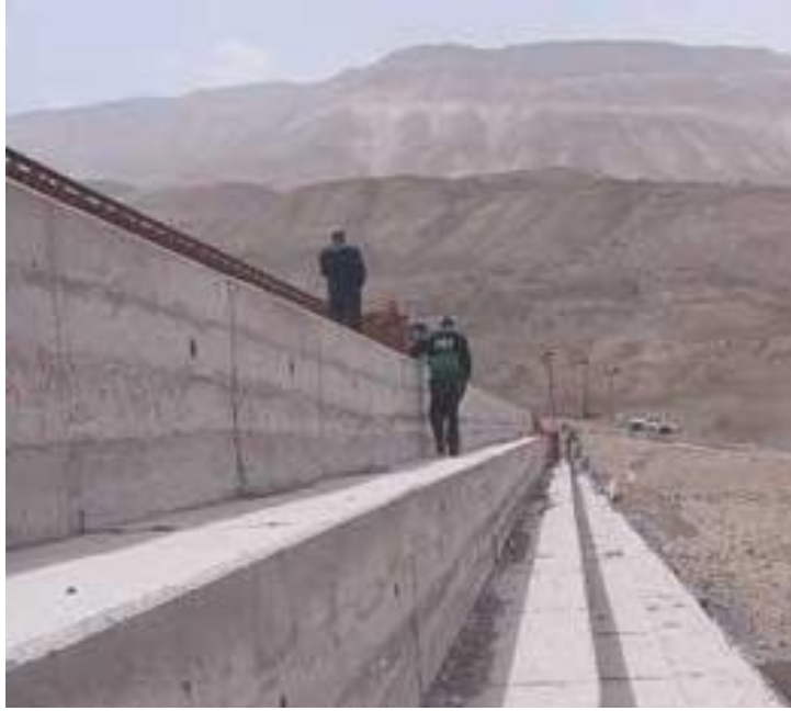
Figure 2.19 Example of layer thickness for a RCCD.
