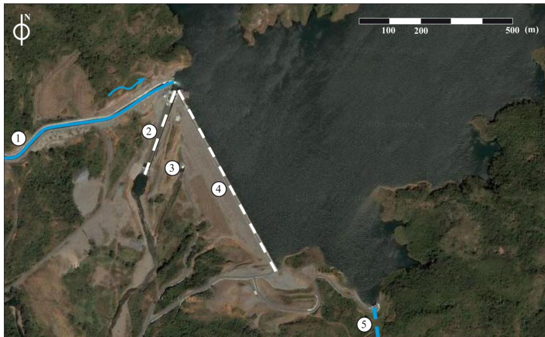
Figure 3.3 Overview of the Barrigon dam area
