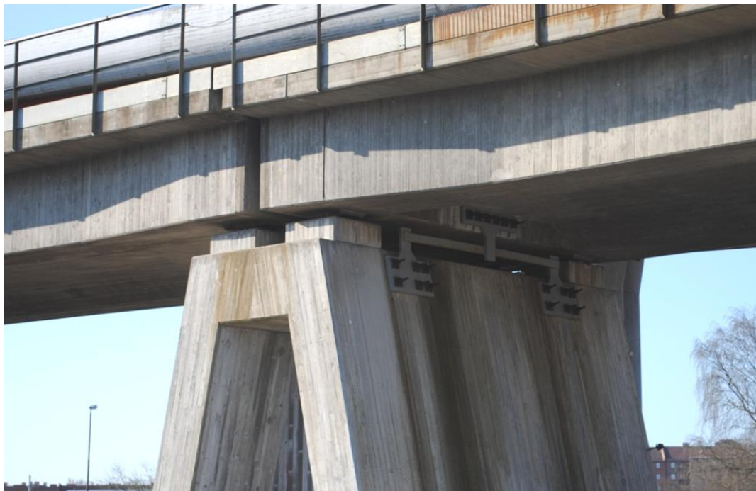
Figure 3.5 Hinge at support 4, bridge Skäran.
