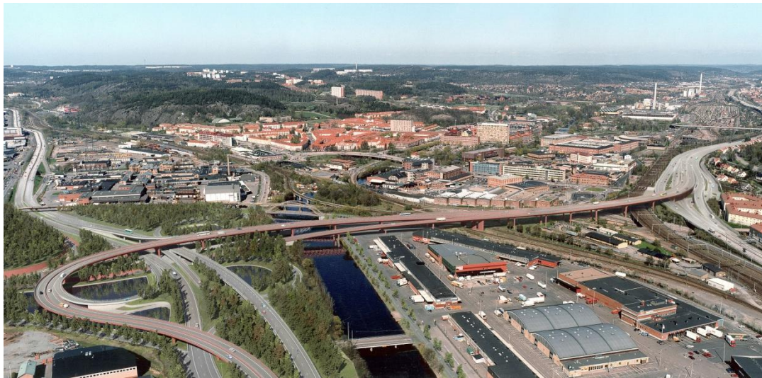
Figure 3.9 Photo montage of Partihallsbron. ( www.trafikverket.se , 2011-05-10, Photo: Per Petersson)
