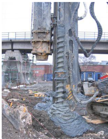
Figure 4.1 Preboring with auger bore. (Photo: Skanska, 28 January 2009)
