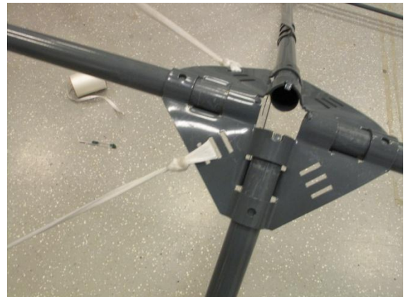
Figure 42 Joint with cross braces
