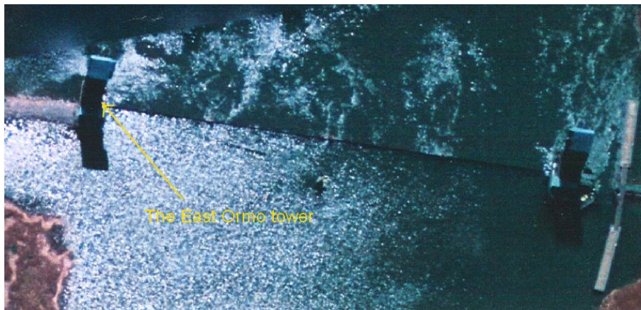
Photo 1 - Ormo's screen facility with damming, downstream view
