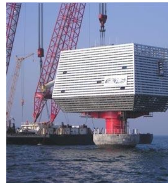
Figure 28 Offshore substation in Rödsand
