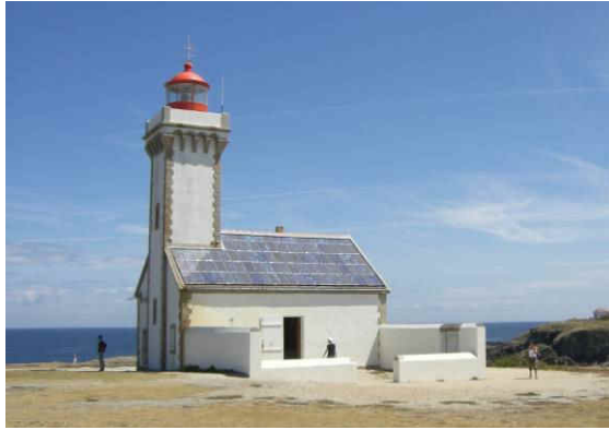
Figure 1-2: Off-grid PV installation on a remote lighthouse in Souzon (Belle Île en Mer - France)
