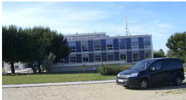
Figure 1-3: Building integrated PV installations at INETI (Lisbon - Portugal).
