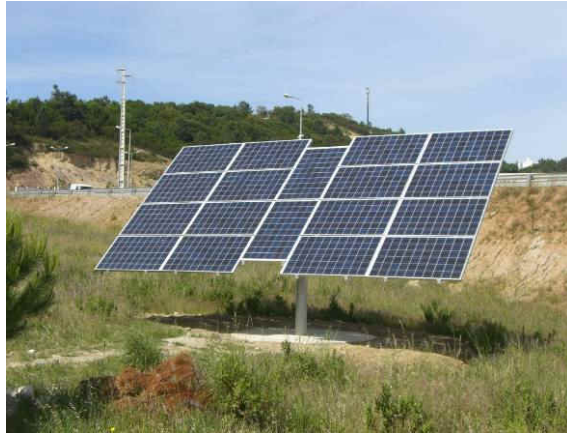
Figure 1-1: On-grid PV installation with tracking system in Venda do Pinheiro (Portugal)
