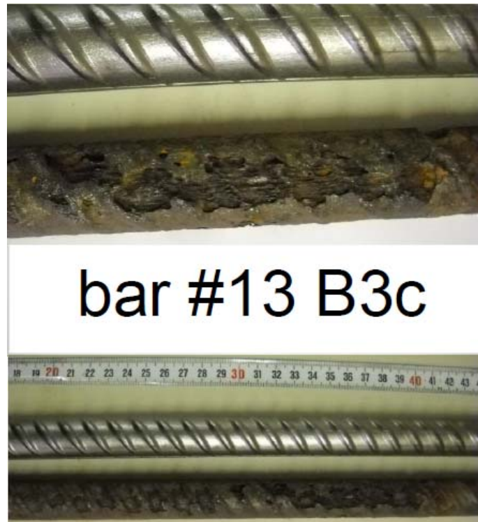
Figure 5.11 (continued): Morphology of the corroded bar surface.
