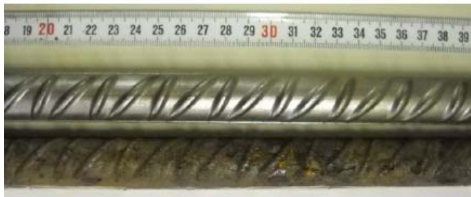
Figure 5.11 Morphology of the corroded bar surface.
