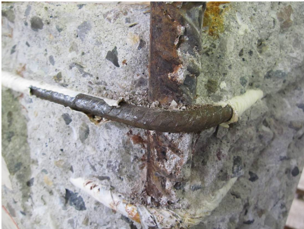
Figure 5.9 Type B specimens: uncorroded stirrup surface, after removing the protection tape.
