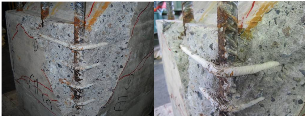
Figure 5.8 The corrosion attack of the main bars from the bottom.
