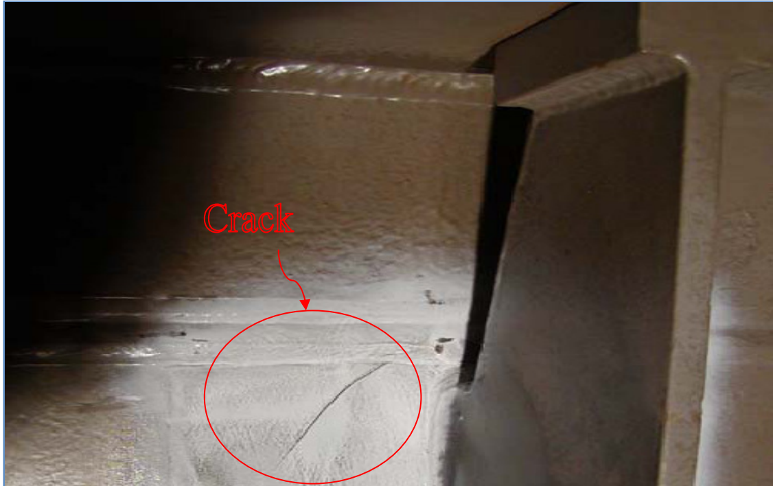
Figure (7-1) the cracks that were discovered in 1990 [17]
