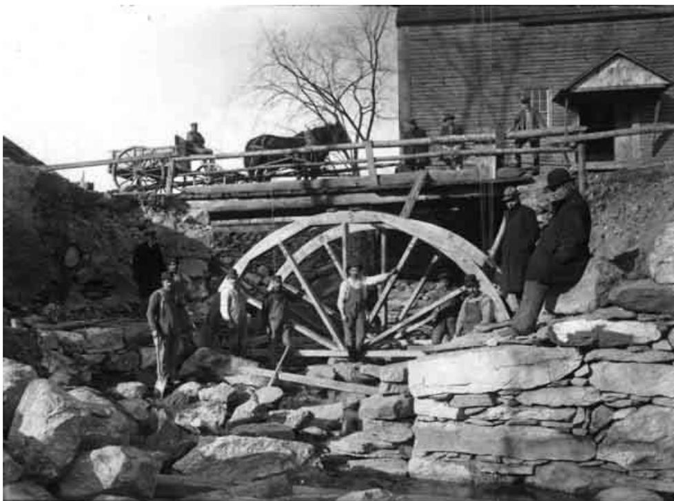
*Figure 3.1 Centering for an unknown bridge in Connecticut. Connecticut's historic highway bridges (2010)*
