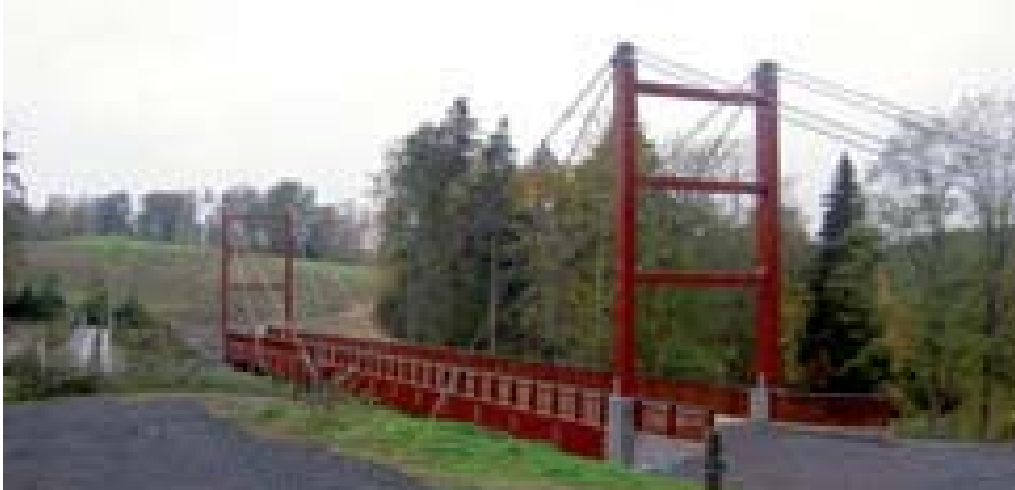
Figure 2.10 Cable stayed timber bridge in Sweden. (Moelven, 2010)
