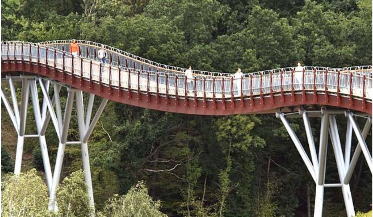
Figure 2.4 "The Dragon's Tail" in the Thuringia region in Germany. The undulating bridge, with 240m length, spans a 25m deep valley close to the town of Ronneburg. (CSCAE, 2010).
