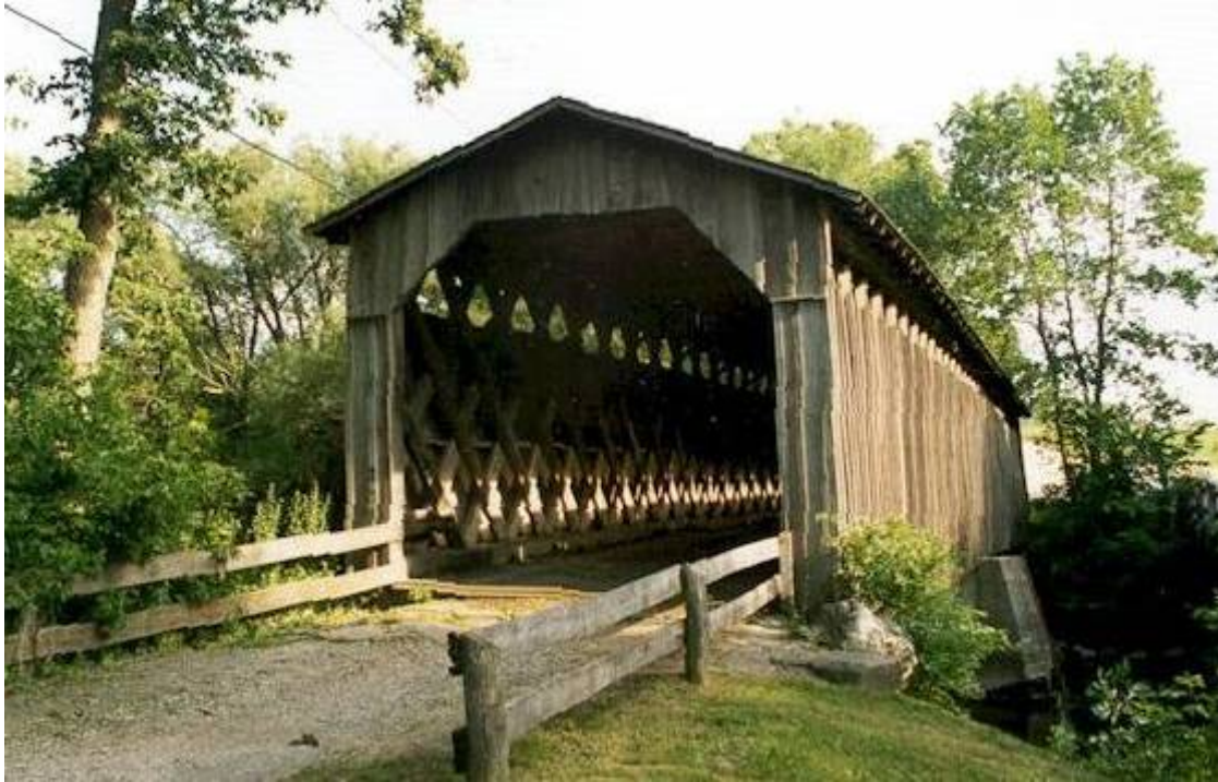
Figure 2.1 Covered bridge built by the Town of Cedarburg, Wisconsin, United States. It was built in 1876 and retired in 1962. Figure courtesy of American Society of Civil Engineers. (Ozaukee County, 2010)
