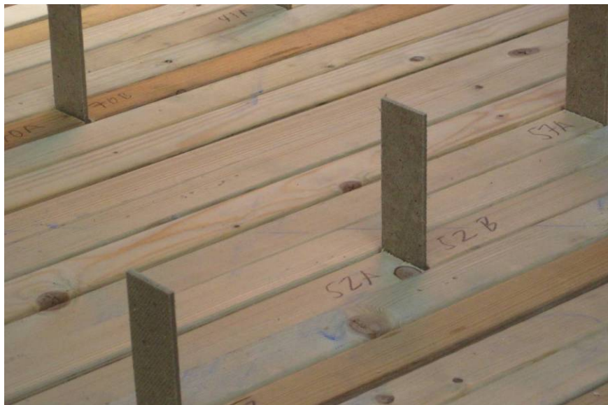
Figure 7.5 Butt joint pattern in the square deck was a 1 in 8 pattern. In this photo thin fibre board plates are used while assembling the deck, in order to make a gap between the two lamination ends.
