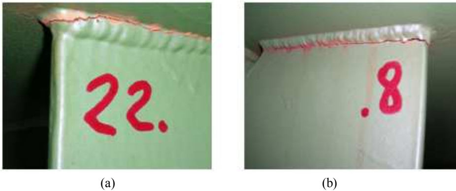
Figure 2.2: (a) root crack; (b) toe crack, Greiner & Taras (2009)
