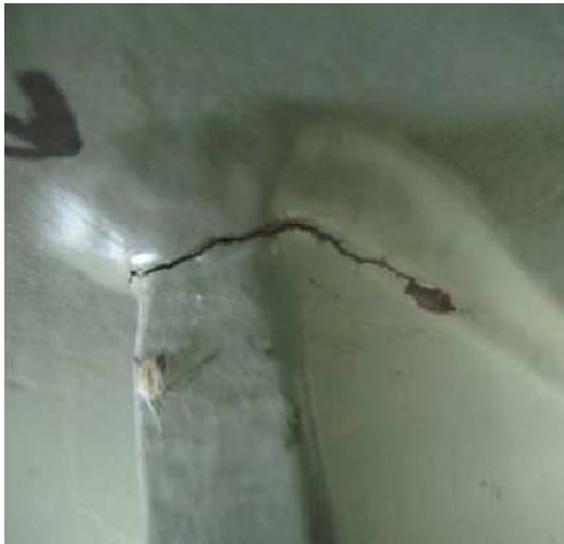
Figure 3.7: Toe crack at a vertical web stiffener, James & Kärrfelt, (2009)
