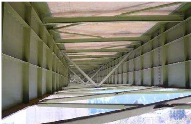
Figure 2.1: Studied bridge by Greiner & Taras, 2009
