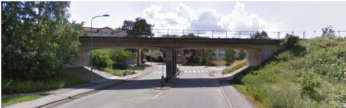
Figure 5.1 Photo of the north side of the bridge over “Sparrmansvägen”.(Google Maps, 2010)
