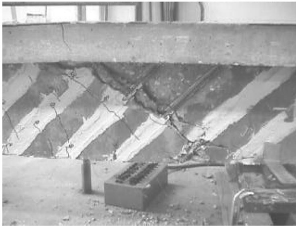
Figure 3.11 Beam with inclined near surface mounted carbon FRP rods after shear failure. (De Lorenzis & Nanni, 2001)
