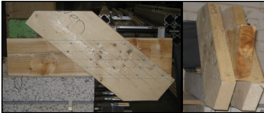
Figure 7.5 Joint from roof truss inspected
