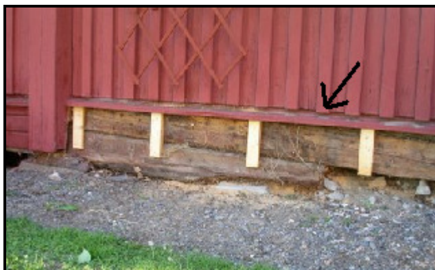
Figure 4.3 Board draining water coming down the wall ( http://hvilaro.blogspot.com/2008/07/byte-av-syllstockar.html , 2009)
