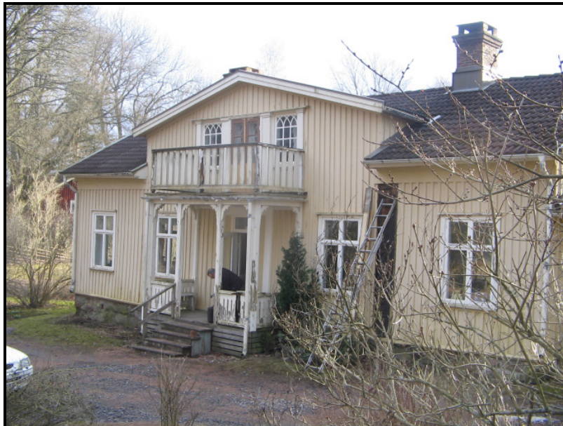
Figure 6.1 Log house inspected with digital radiography
