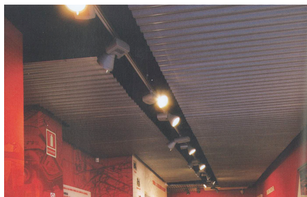
Figure 2.6 Track bound spotlights
