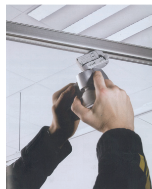
Figure 2.7 Mounting a track bound spotlight
