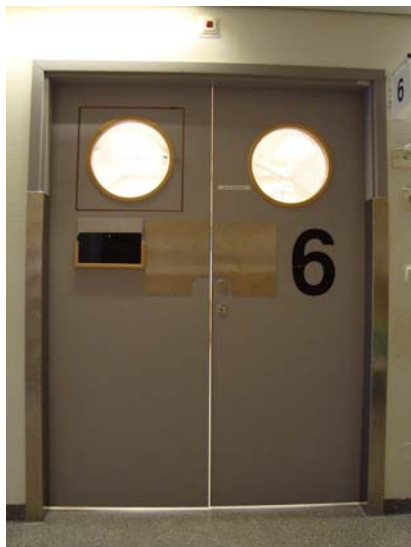
Figure 3.3 Door into the operating room seen from the corridor.
