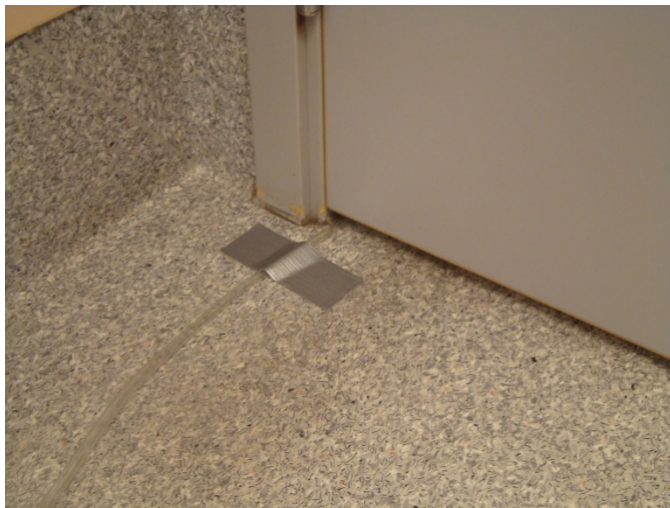
Figure 5.6 The second plastic tube connected to the Differential Pressure Transmitter passes the secondary barrier under the door to the corridor.
