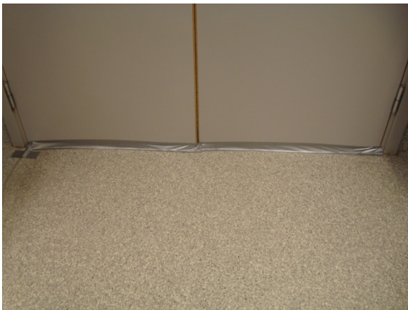
Figure 5.8 Air gap between doors and floor blocked with duct tape to investigate the gap's consequences on the pressure difference.
