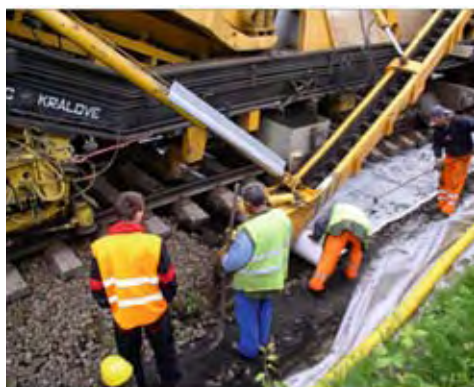
Figure 4.2.3-3: Old ballast removal with geocomposite installation
