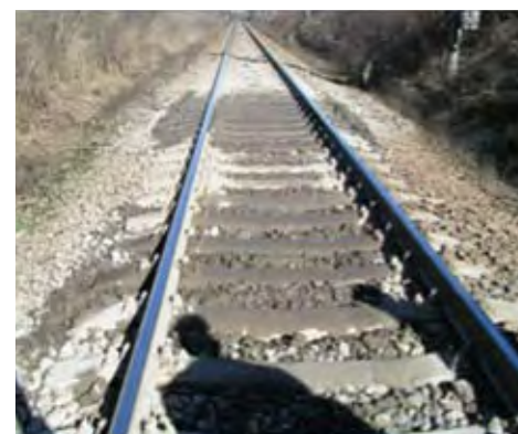
Figure 4.2.3-1: Track with drainage defects before reparation
