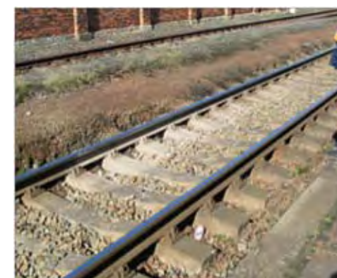
Figure 4.2.3-2: Station track with clear drainage defects
