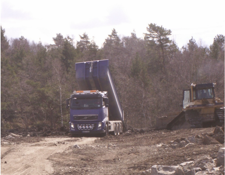
Figure 2-2: dumping dirt at a landfill
