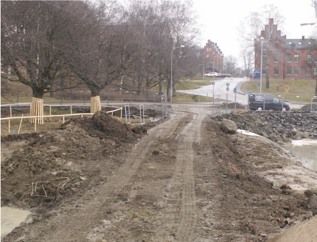
Figure 5-12: soft and muddy terrain on a construction site
