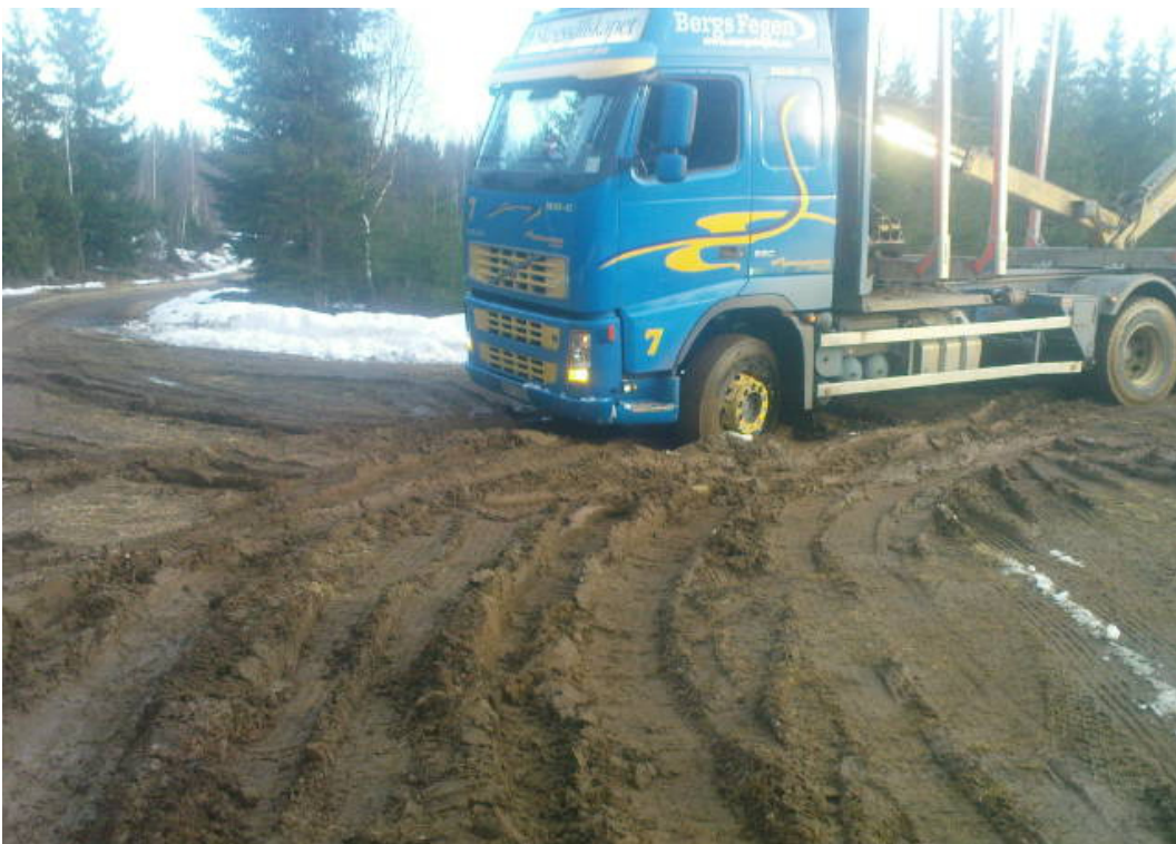
Figure 5-15: deep mud after heavy rain on forest road
