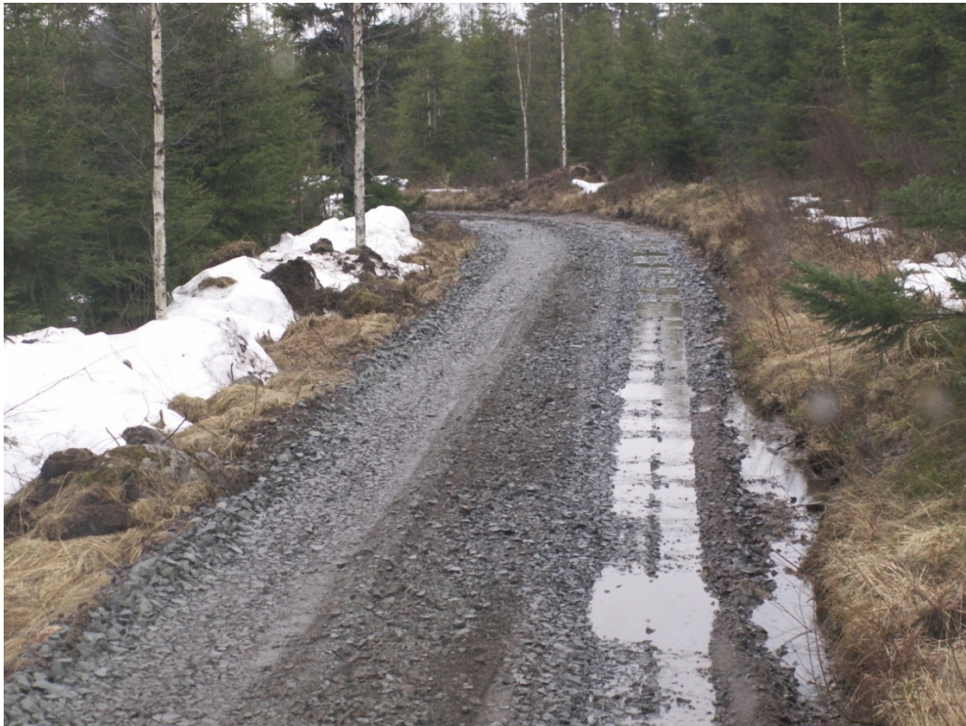
Figure 5-16: uneven forest road
