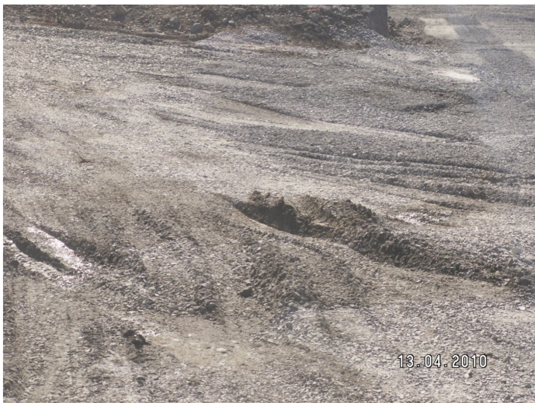
Figure 5-9: deep tracks on construction site
