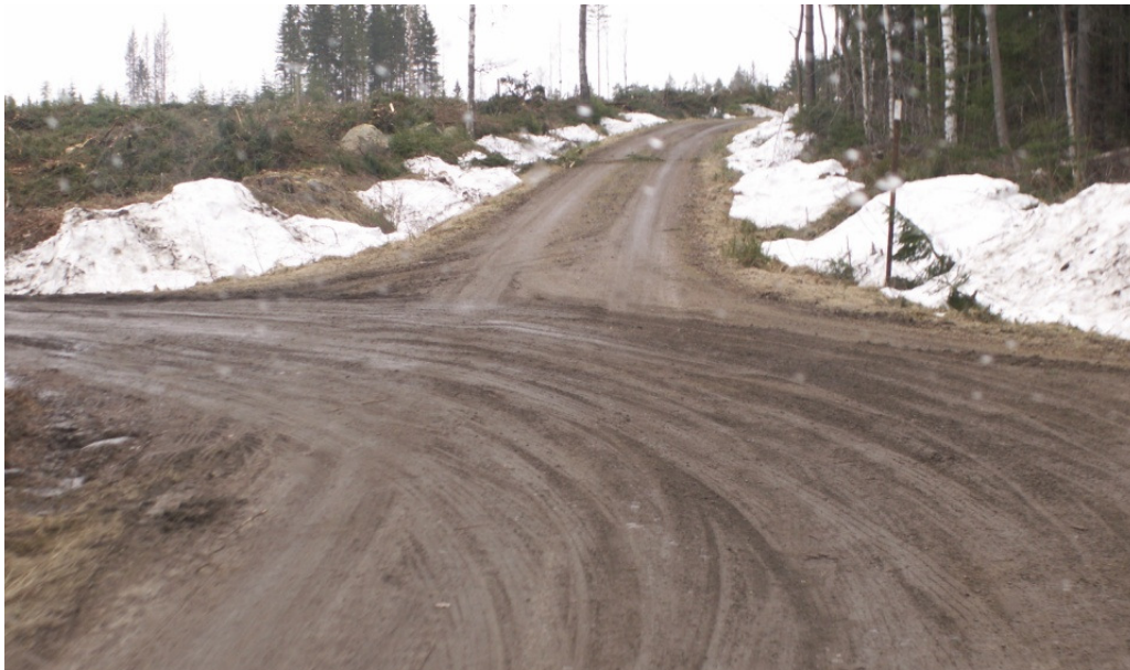
Figure 5-31: slight slope on a forest road, ice forming as temperature falls
