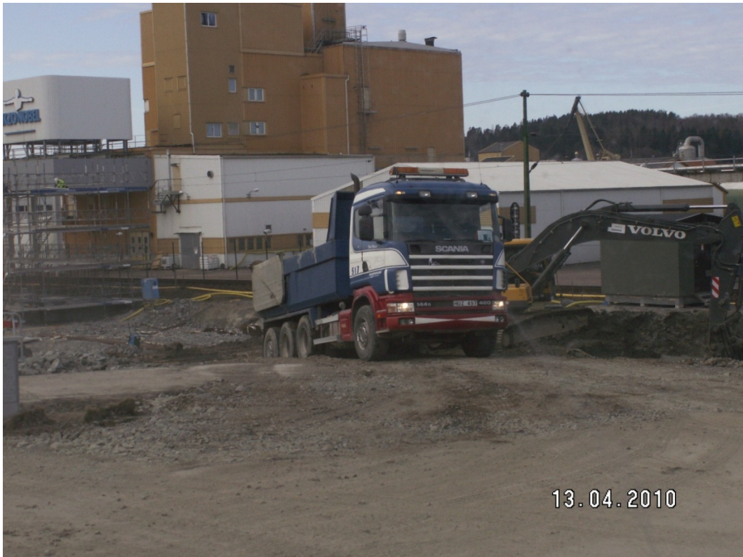
Figure 5-18: steep slope on construction site
