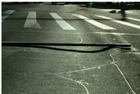
Figure 3.2 A picture illustrating a rut (PCA 2010).
