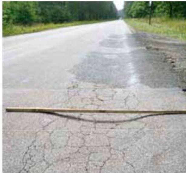
Figure 2-9 Rutting in the unbound layer (Kolisoja & Dawson 2006)
