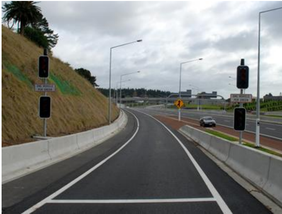
Figure 3.2 Ramp meter with one lane, on a freeway with left hand traffic. (Auckland Motorways)
