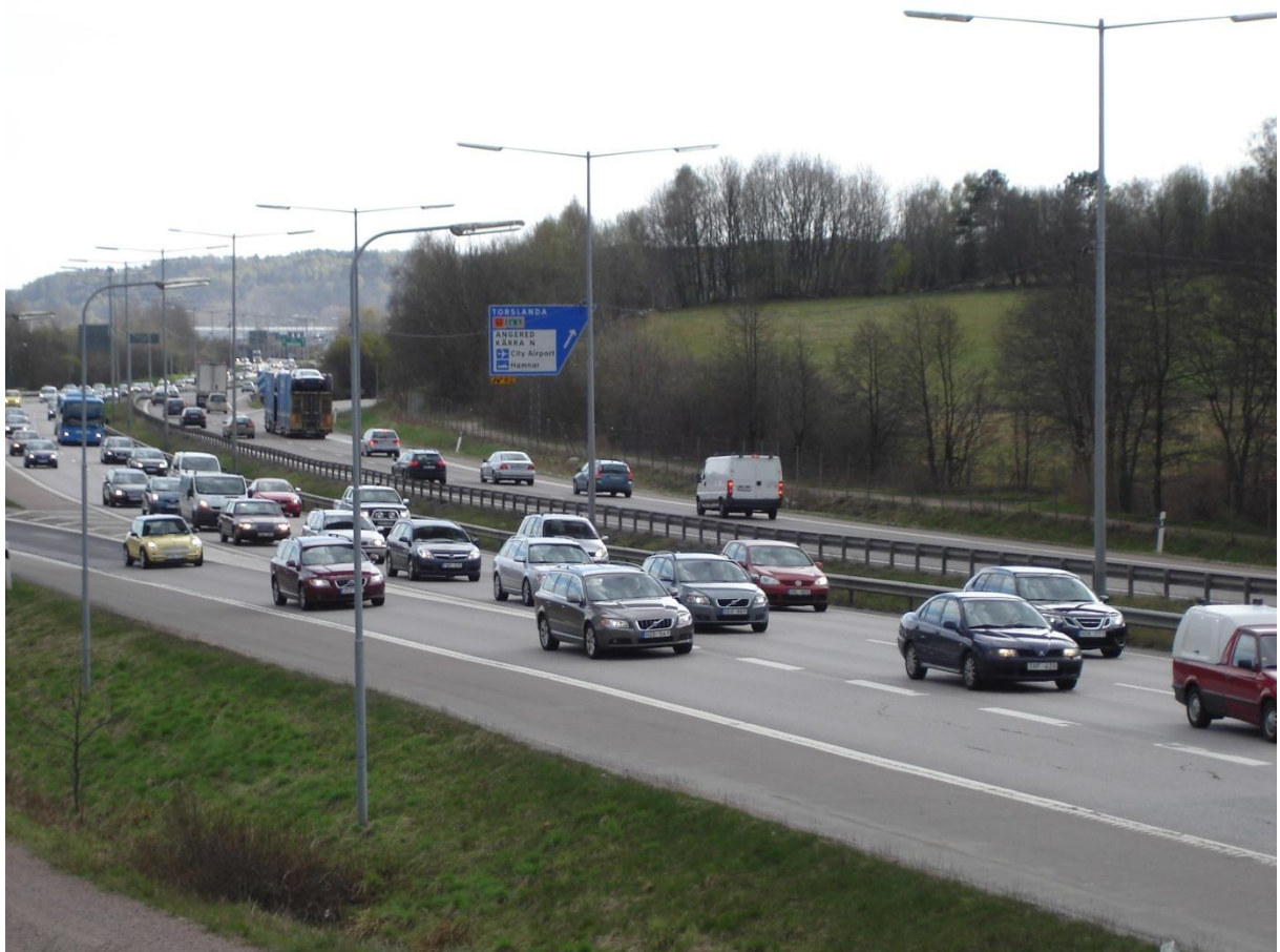
Figure 3.6 Klareberg junction close to the northbound on-ramp.
