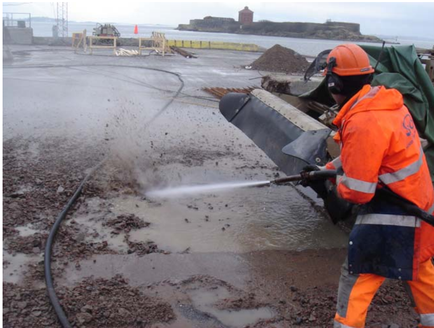
Figure 9.13 Cleaning the Surface 1 taking away the rubble.
