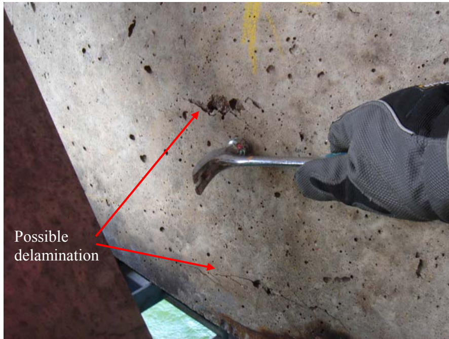
Figure 9.28 Hitting with the hammer to find the possible delamination.
