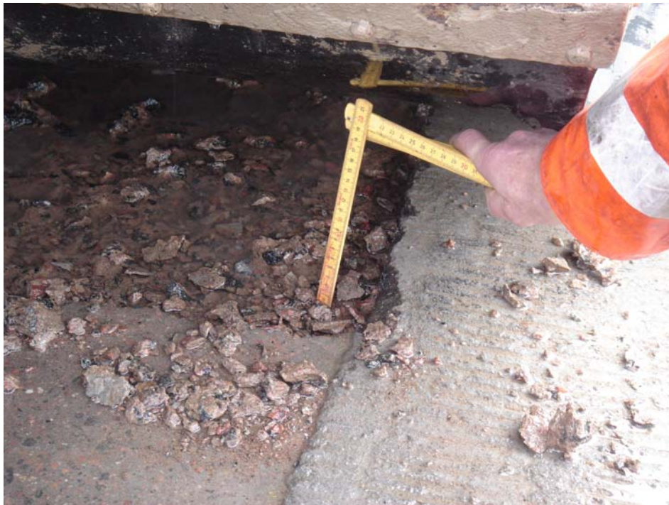
Figure 9.12 Checking the depth after the first waterblasting.
