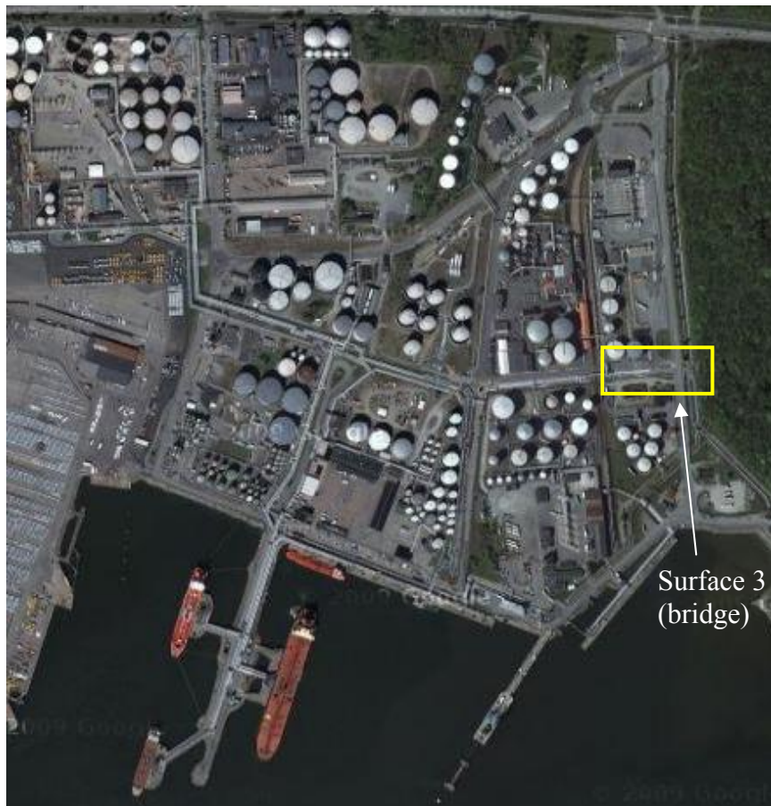
Figure 9.33 Skarvikshamnen with the emplacement of the bridge marked.
