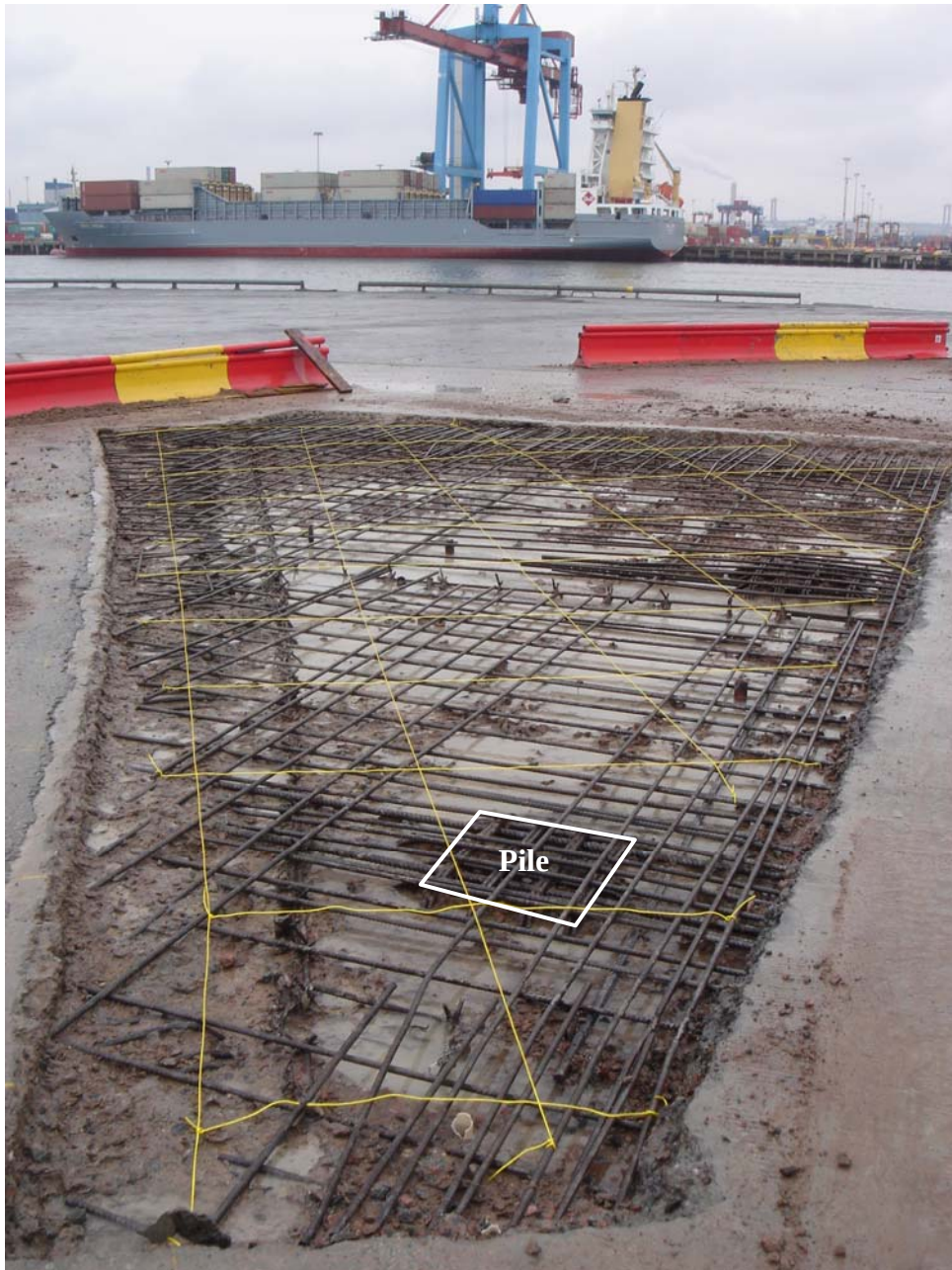
Figure 9.16 Grid at the Surface 1 waterblasted with one pile marked.
