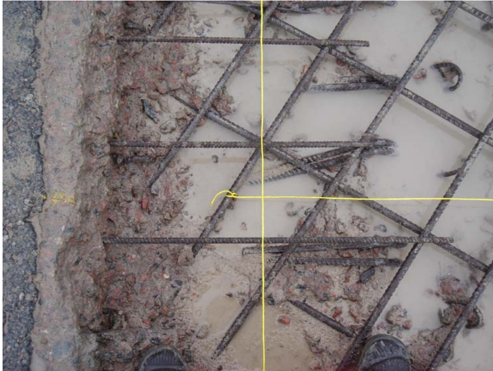
Figure 9.20 Test point L1M7 of the beam. No corrosion damages detected.
