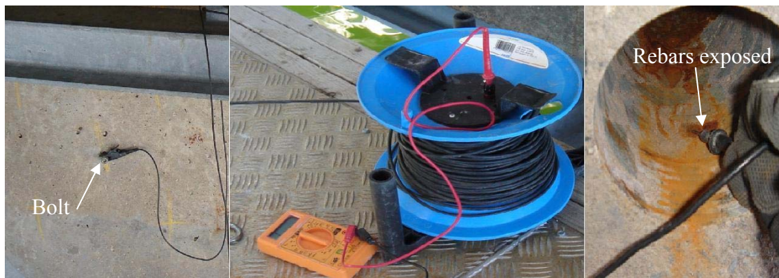
Figure 7.6 Checking the connectivity of the beam at Torshamnen.
