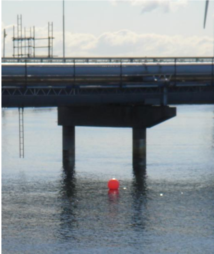
Figure 9.23 Position of the Surface 2 in the bridge.
