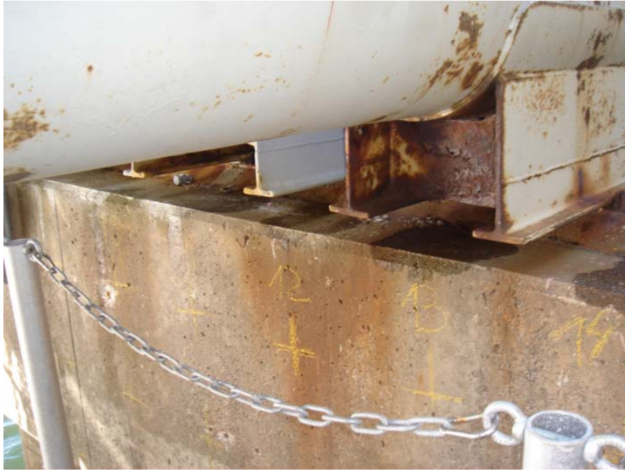
Figure 9.29 Testing the side C. The supports of the pipelines prevent some tests.
