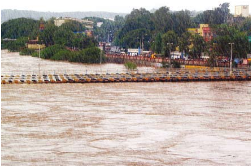
Annual flooding during Monsoons render some bridges unsafe for vehicular usage.
