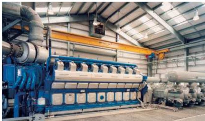
*Figure 2-1: The Wärtsilä 34SG engine. By courtesy of Wärtsilä [2] [3] [4]*
