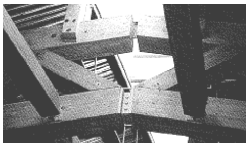
Figure 5.4 Example of connection at the crown in the lower chord, MOELVEN brochure
