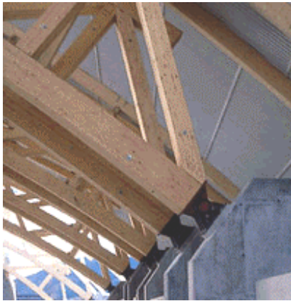
Figure 5.3 Abutment connections, Håkons Hall in Lillehammer, Carling, Svenskt limträ AB (2001)
