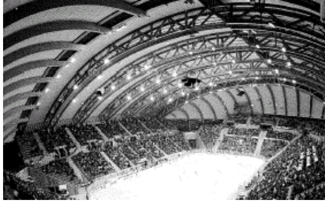
Figure 3.33 Håkons hall, Lillehammer – Notice the absence of lateral bracing in the lower chord
