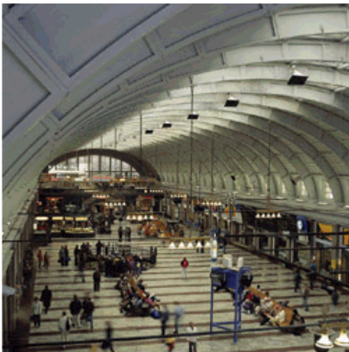
Figure 1.1 Hall of the central station in Stockholm, Carling, Svenskt limträ AB (2001)
