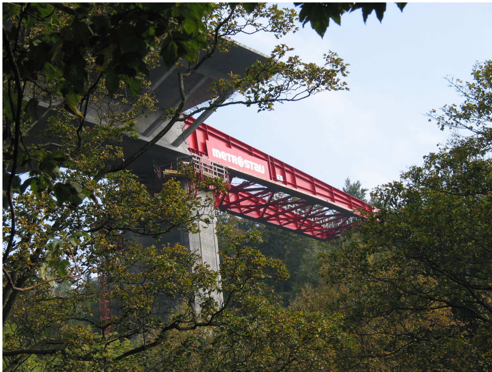
Figure 4.1 Launching nose used during launching of the Rybný Potok bridge.
