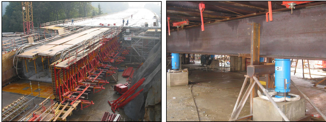
Figure 3.7 Left: View of the casting yard. Right: The steel grid is resting on hydraulic jacks.
