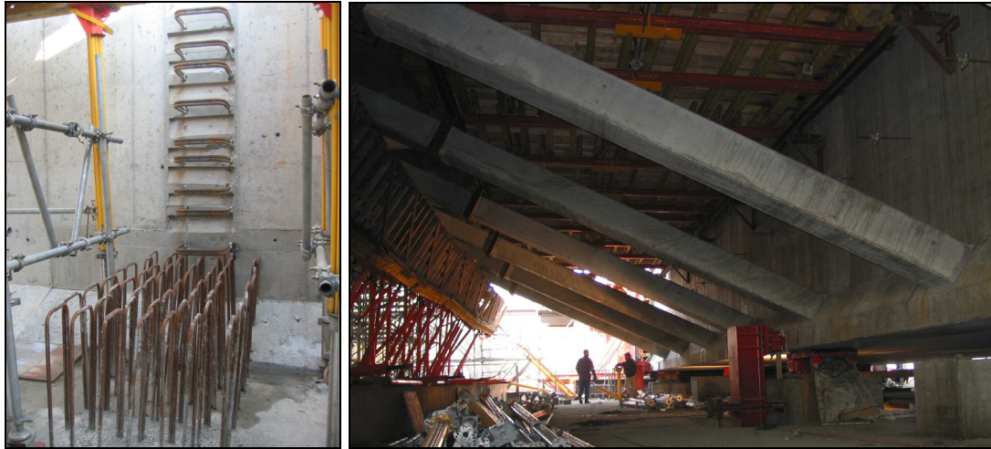
Figure 3.8 Left: Reinforcement for heels assembled in the casting yard. Right: The diagonal struts between the box and deck of the superstructure.
