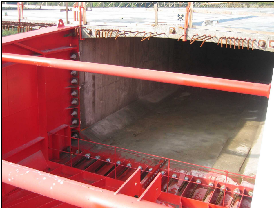
Figure 3.11 Top: The launching nose. Bottom: The joint between the launching nose and the superstructure.
