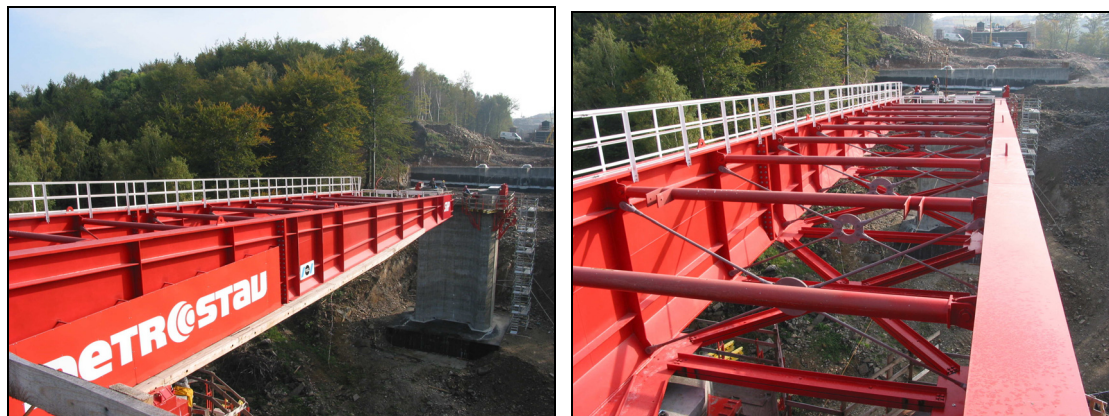
Figure 4.2 Example of launching nose with I-beams.
