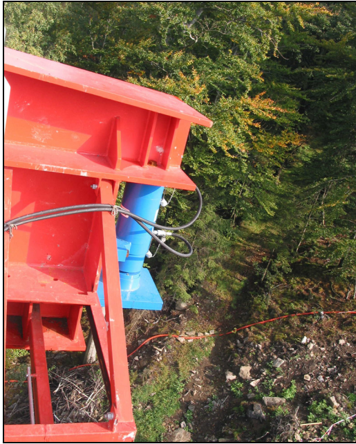
Figure 4.4 Hydraulic jack integrated in the launching nose.
