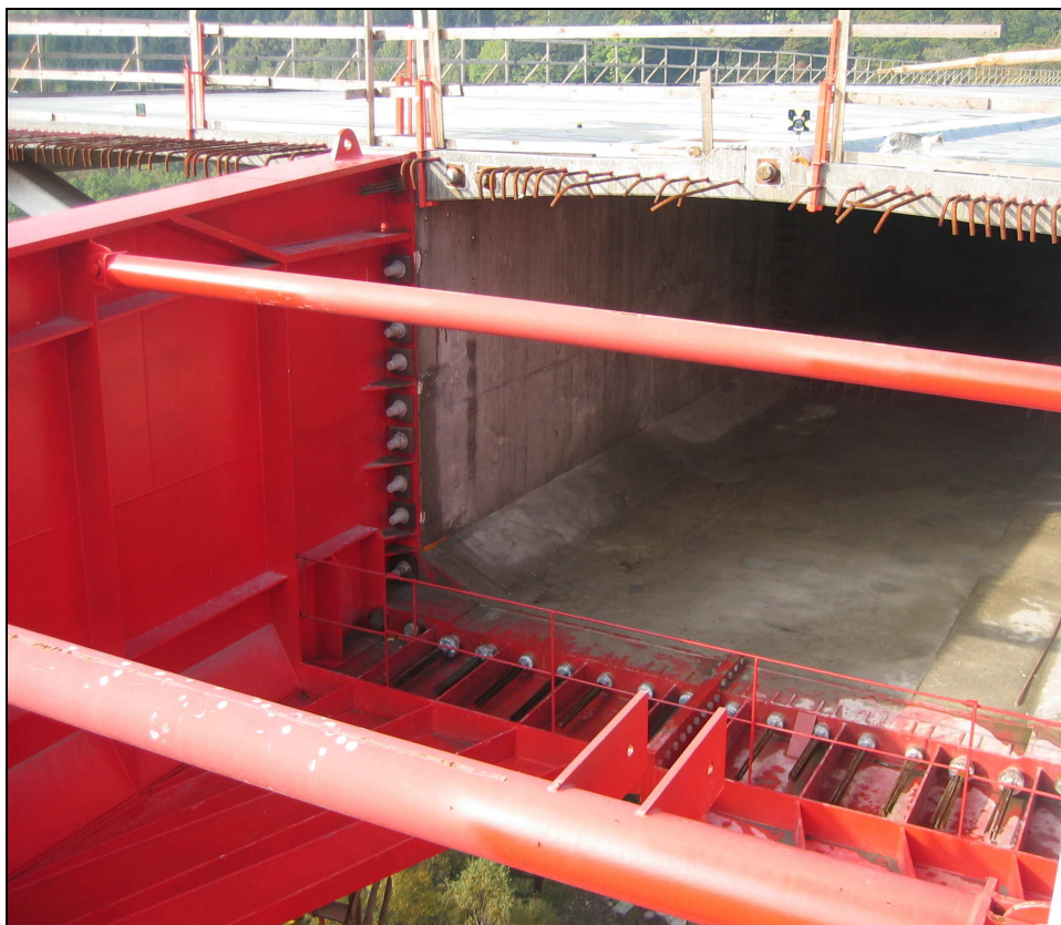
Figure 4.3 Joint between the launching nose and the box girder.
