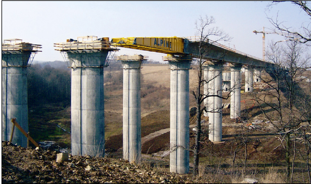
Figure 2.4 Launching nose during erection of the Gebergrund bridge in Germany (Doka 2003).
