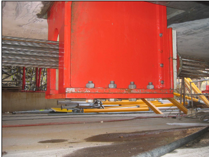
Figure 3.10 Steel brackets mechanically attached to the concrete segment. The steel tendons pulling the bridge forward during launching are also visualised.
