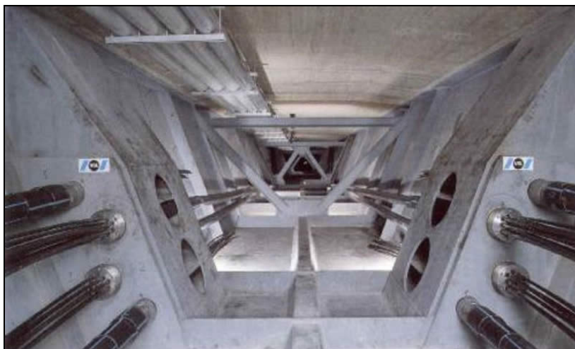
Figure 5.2 External prestressing inside a box girder (VSL Constructions Systems).
