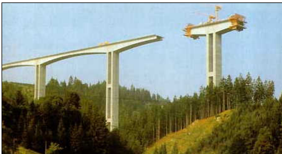
Figure 2.3 Balanced cantilever construction, "Lavanttal bridge" (TDV 1984).
