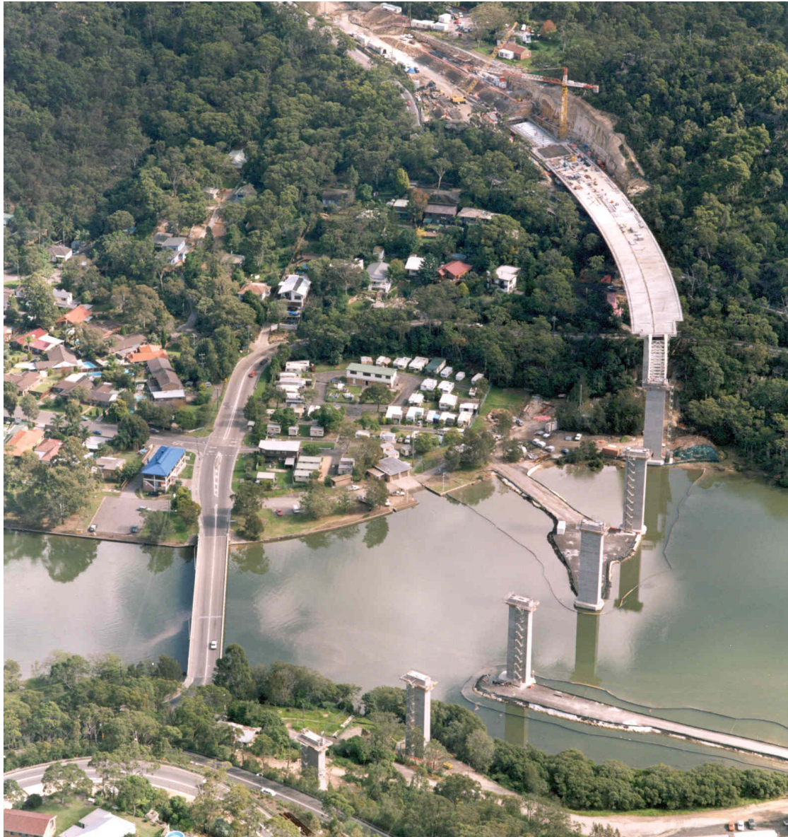
Figure 4.1 Launching of the Woronora Bridge in Australia. Radius of curvature was 460 m, launching downwards with 6,0% slope and the superstructure had a total weight of 20 000 tons. Typical span length 58,7 m. (Courtesy VSL)
