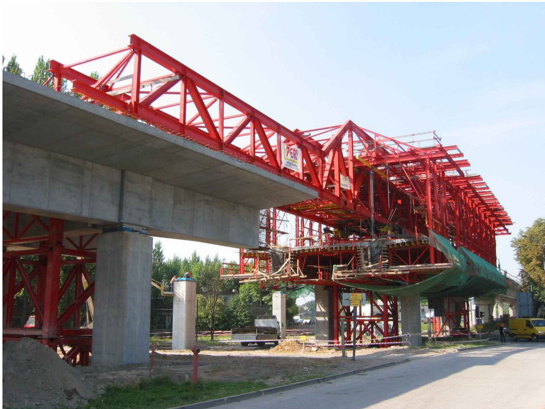
Figure 4.3 Construction of a concrete bridge with a travelling gantry. In this specific case the height of the bridge is quite low, why the risk of working at the gantry is limited. However, when constructing with the IL method almost no high level work is needed. (Courtesy Skanska SA Poland (2002))
