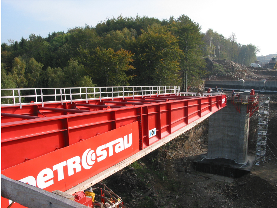
Figure 8.15 View of launching nose and the final pier in front of the end abutment.
