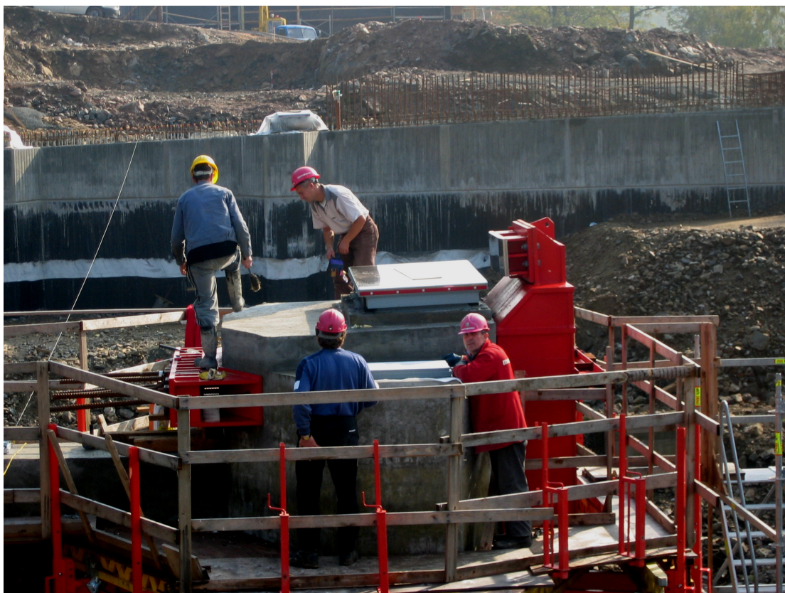
Figure 1.14 Preparation of a sliding bearing at the Rybny Potok Bridge.
