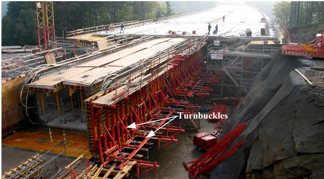
Figure 8.8 Formwork of the Rybny Potok Bridge. Notice the turnbuckles by which the formwork was manually mechanically moved to the side.
