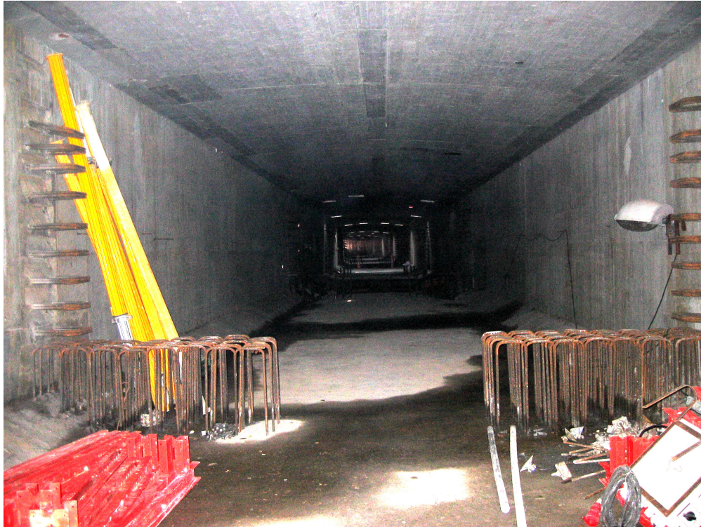
Figure 8.6 Reinforcement for deviators used for the external polygonal tendons.
