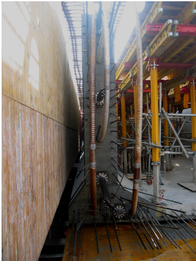
Figure 1.5 The bottom slab and the webs have been cast and the formwork is moved. The inner formwork for the top slab is being mounted inside the box (to the right in this picture).
