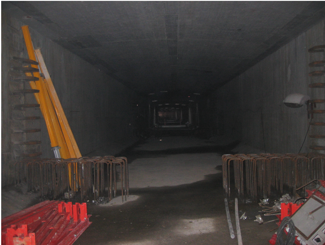
Figure 6.5 Picture from inside a box girder where the reinforcement for two concrete deviators is seen. The deviators will be cast when the bridge is totally launched.
