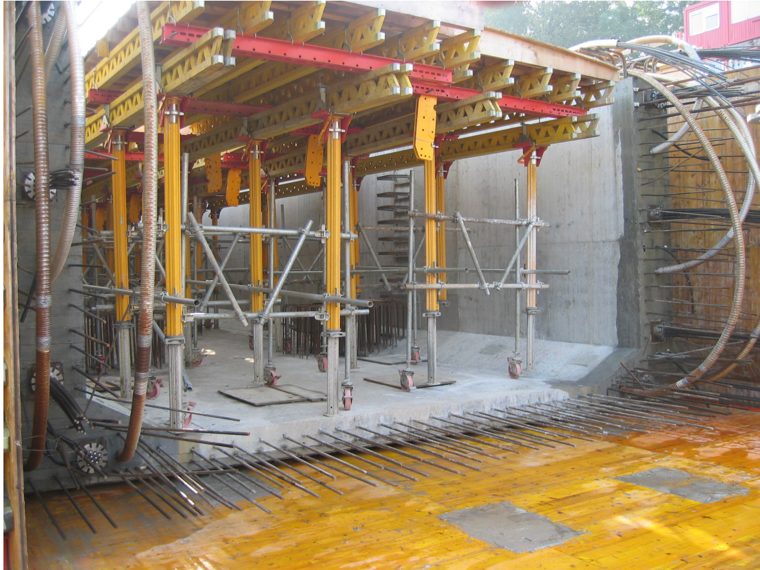
Figure 8.4 Rybny Potok Bridge section. Notice the tensioned prestressing anchorages and the continuous tendons that are to be tensioned after the completion of the next segment.
