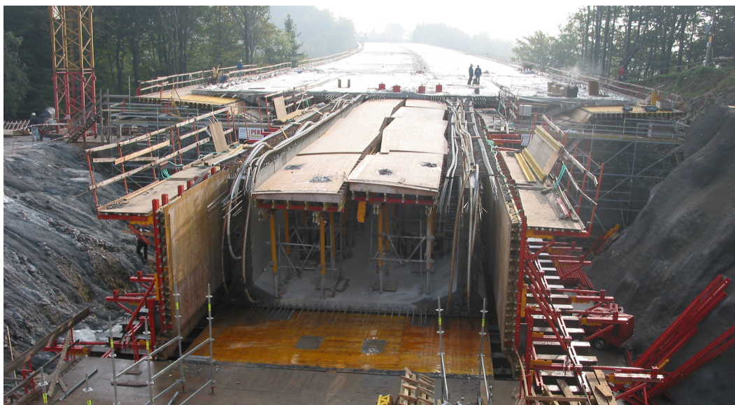
Figure 1.1 View over the casting yard and the bridge deck at one abutment of the Rybny Potok Bridge.
