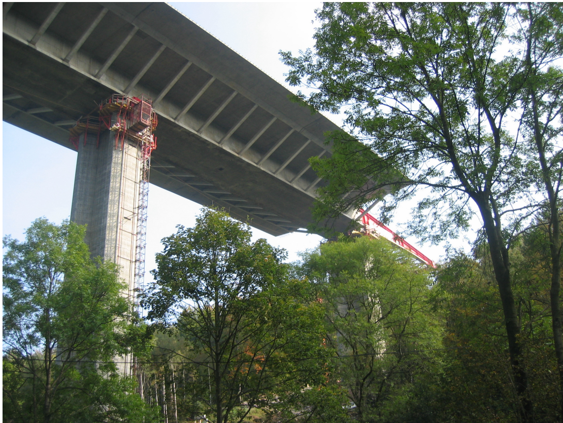
Figure 1.2 The incremental launching method provides advantages when it comes to crossing obstacles, in this case a deep valley in Czech Republic.
