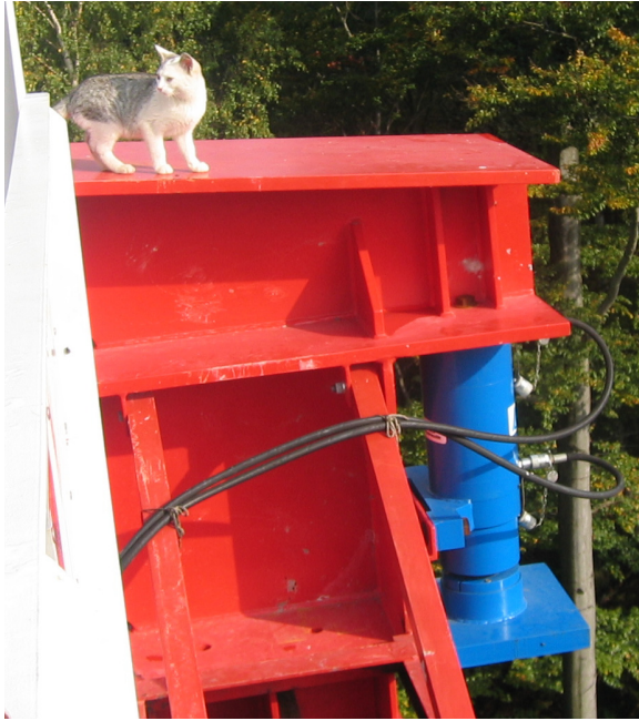
Figure 8.13 Lifting jack in front of the nose.
