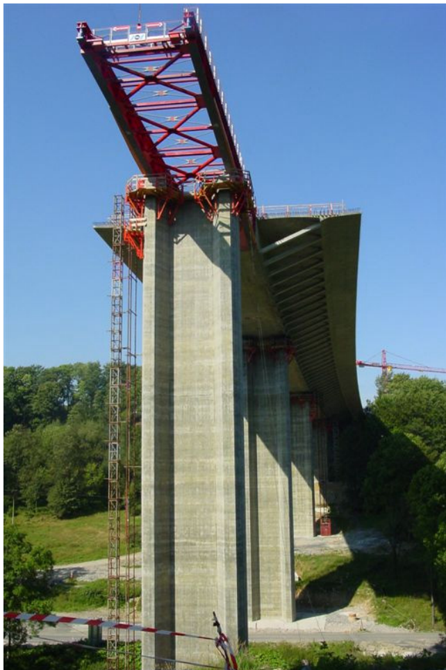
Figure 8.1 Front view of the Rybny Potok Bridge under construction.
