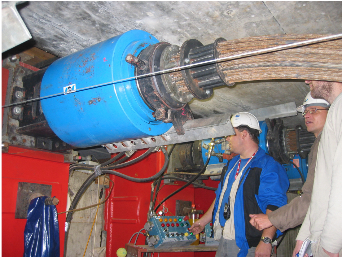
Figure 1.10 A pulling jack. The steel strands are connected to the bridge section 20 m to the left of the jack in this picture, and the jack pulls the strands towards it. The launching direction is to the right.
