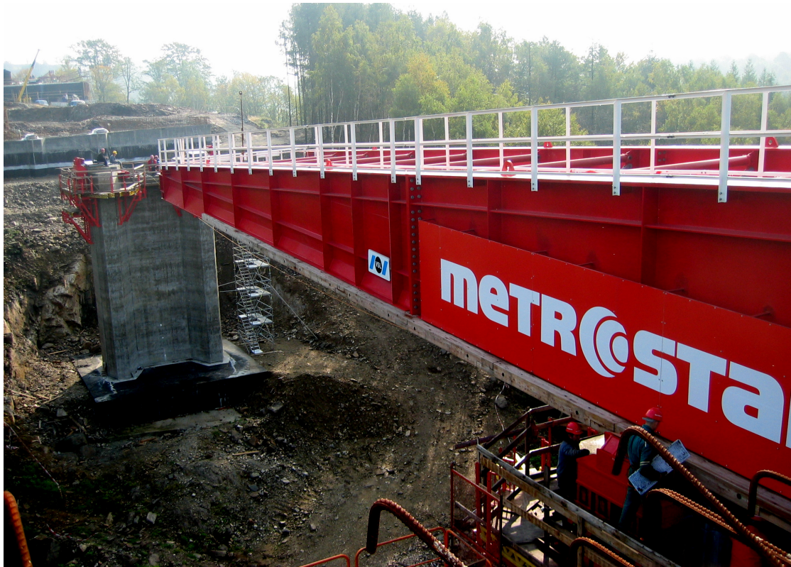
Figure 1.15 The launching nose used for the Rybny Potok Bridge in the Czech Republic. Height of the nose is 4,2 m at the concrete connection and 1,0 m at the front end. The nose is 10 m wide The length of the nose is 36 m.
