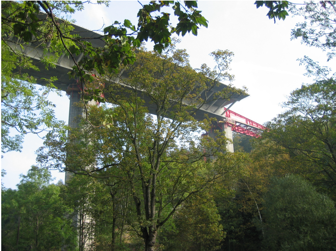
Figure 4.2 One of the main advantages with the IL method is that a bridge can be erected where no scaffolding is possible or economical to build. In this picture the Rybny Potok Bridge is crossing a 40 m deep valley.
