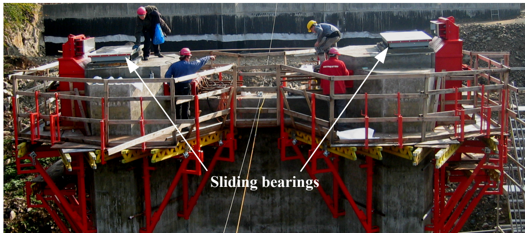
Figure 8.12 Preparation of the sliding bearings on one pier at the Rybny Potok Bridge
