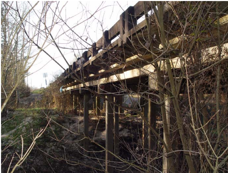
Figure A.1 Lateral view of the White Bayou Bridge.
