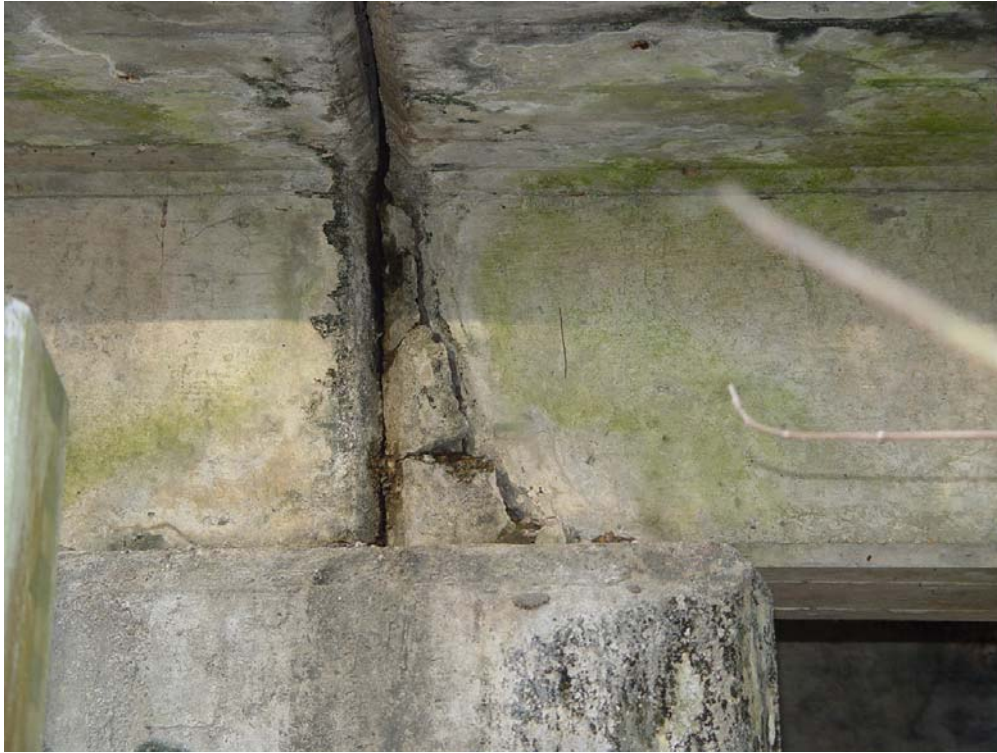
Figure A.7 Detail view of a deteriorated joint.
