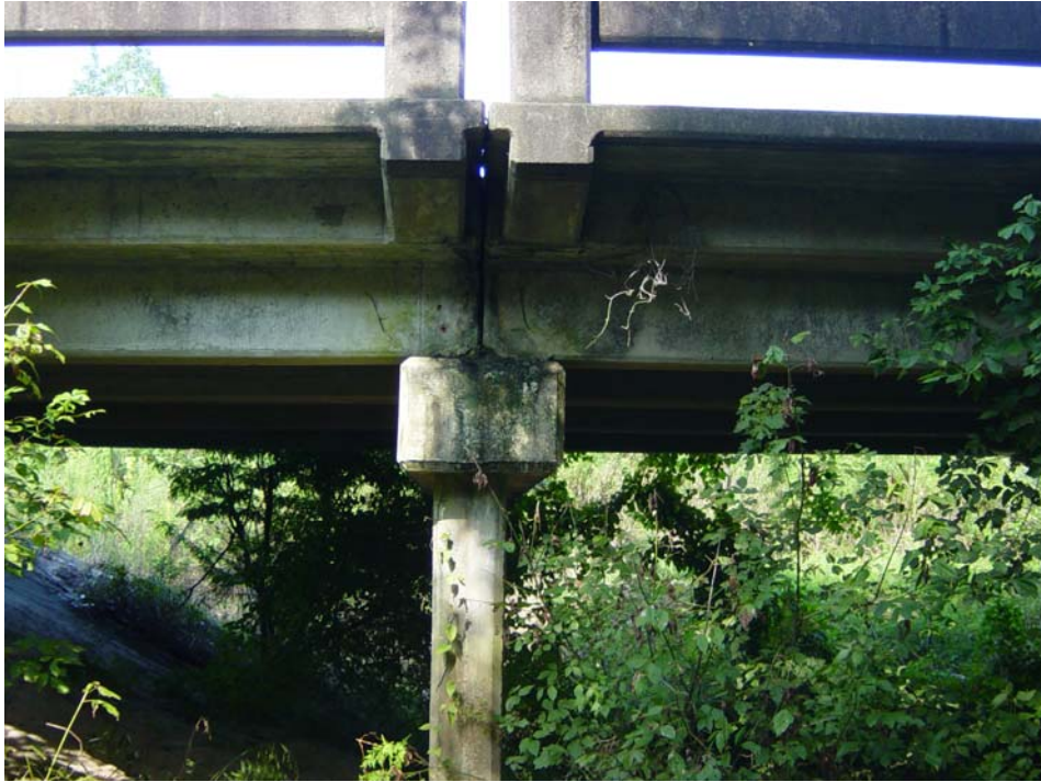
Figure A.3 Joint between spans.
