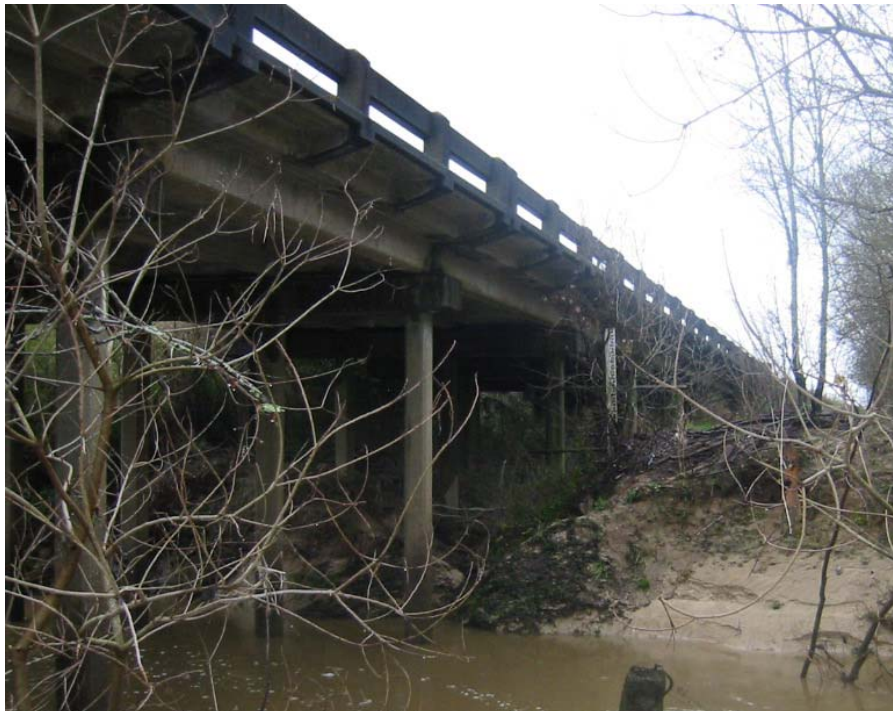
Figure 4.3 Lateral view of the White Bayou Bridge.
