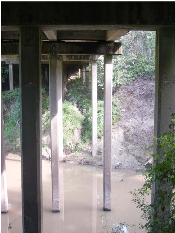
Figure A.2 Bottom view of the White Bayou Bridge (scour can be seen on the piles).
