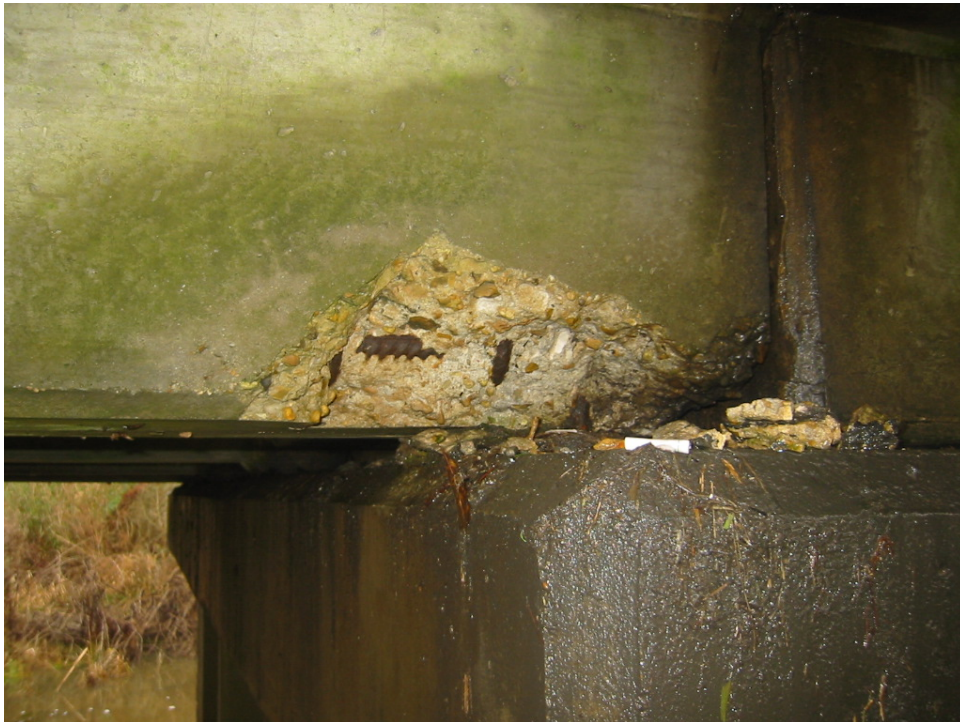
Figure A.6 Detail view of a deteriorated beam.
