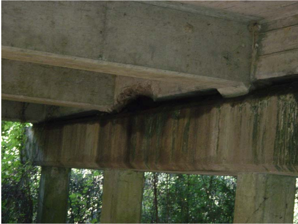
Figure A.5 Bottom view of the concrete spalling deck.
