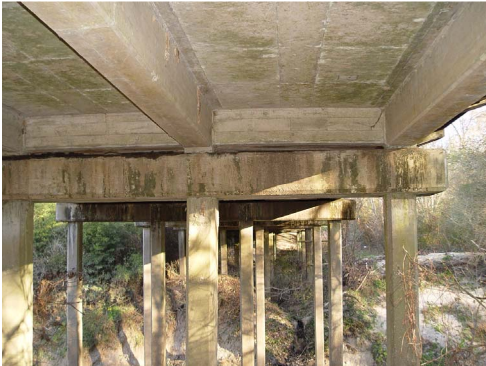
Figure A.4 Bottom view of the bridge deck.
